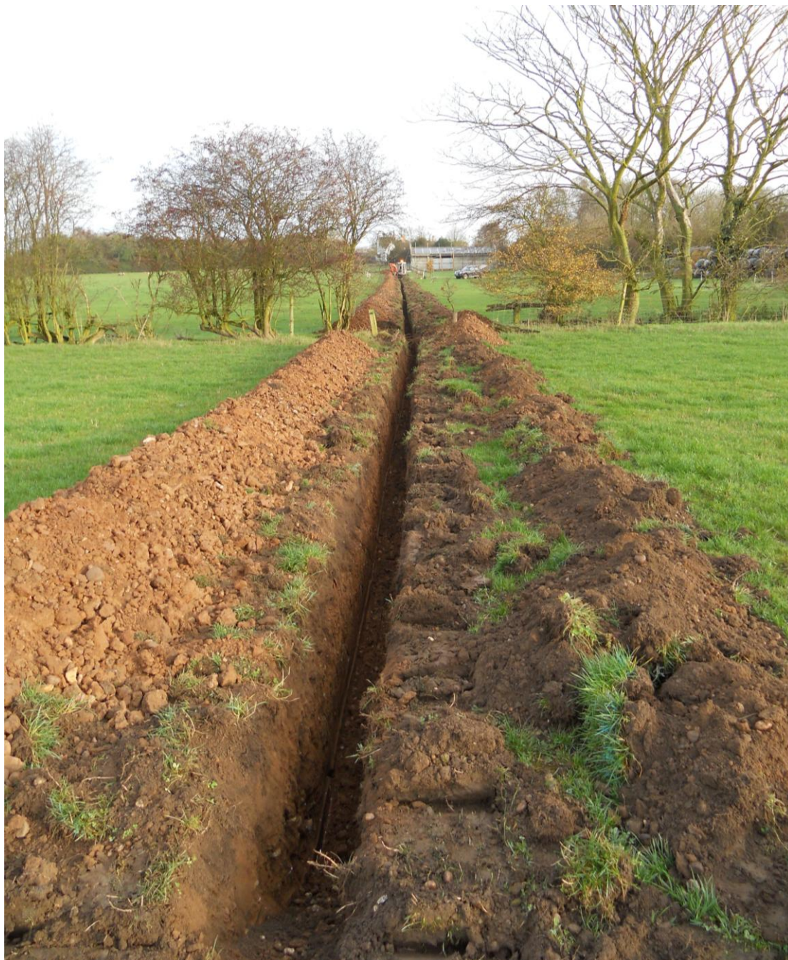
Figure 8. Field 2 looking north towards Field 1
