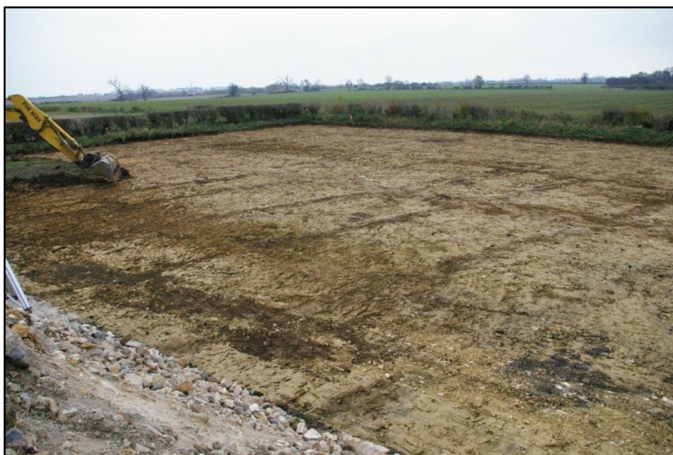
Plate 1: Machine stripping and reducing ground levels
