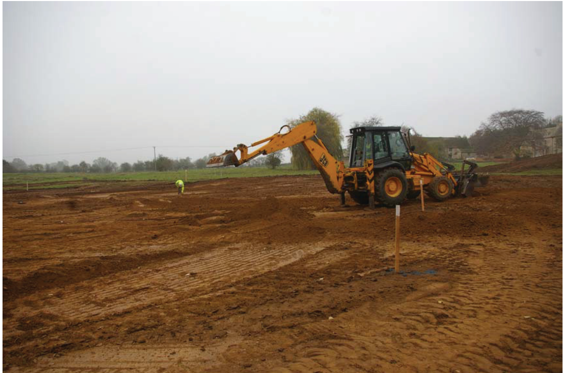
Plate 1: Working progress with JCB, looking south-west
