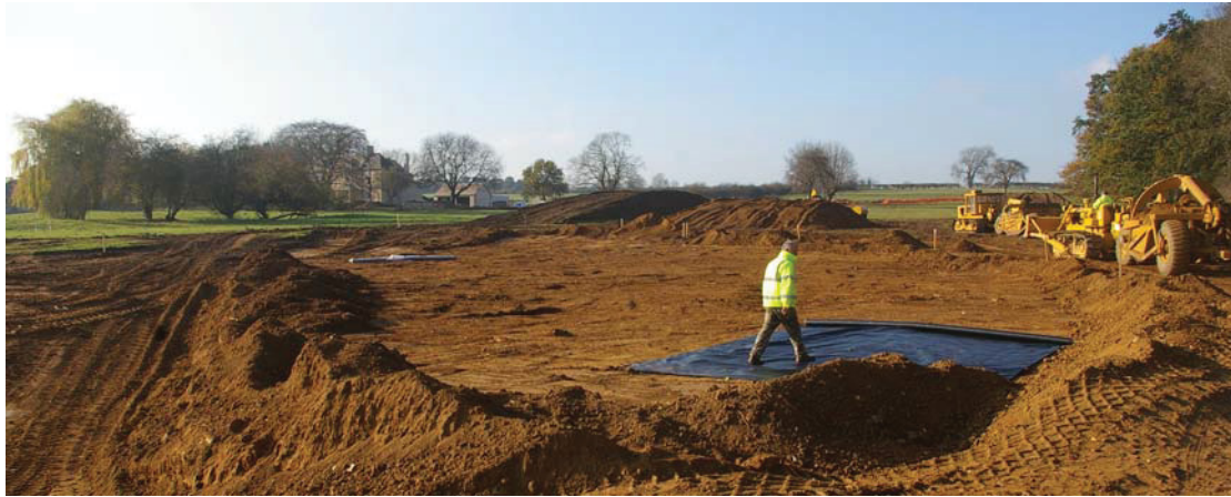
Plate 7: Work in progress on geotextile laying, looking south-west
