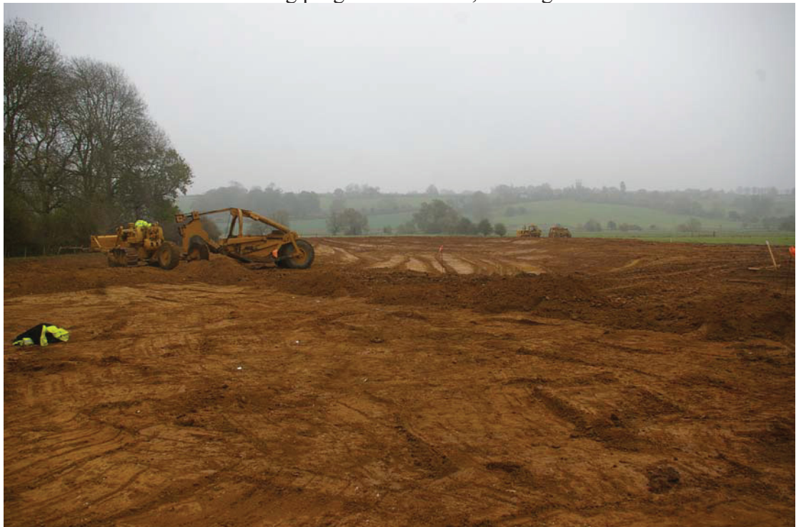
Plate 2: Work continuing on eastern area with box scraper, looking east
