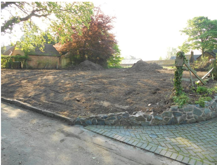
Figure 3: Site after topsoil removal, from Wood Lane looking SE.
