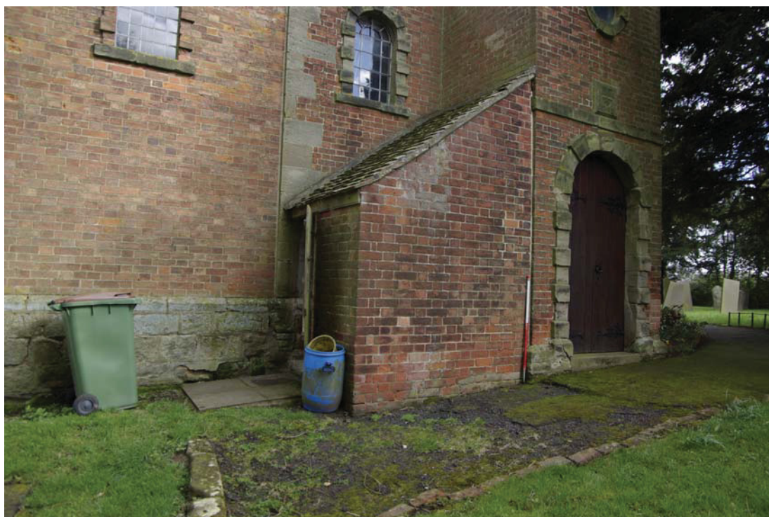
Figure 10. External 19th century store, proposed for demolition. Looking south-east.
