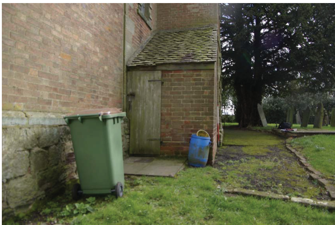
Figure 11. As above, looking south.
