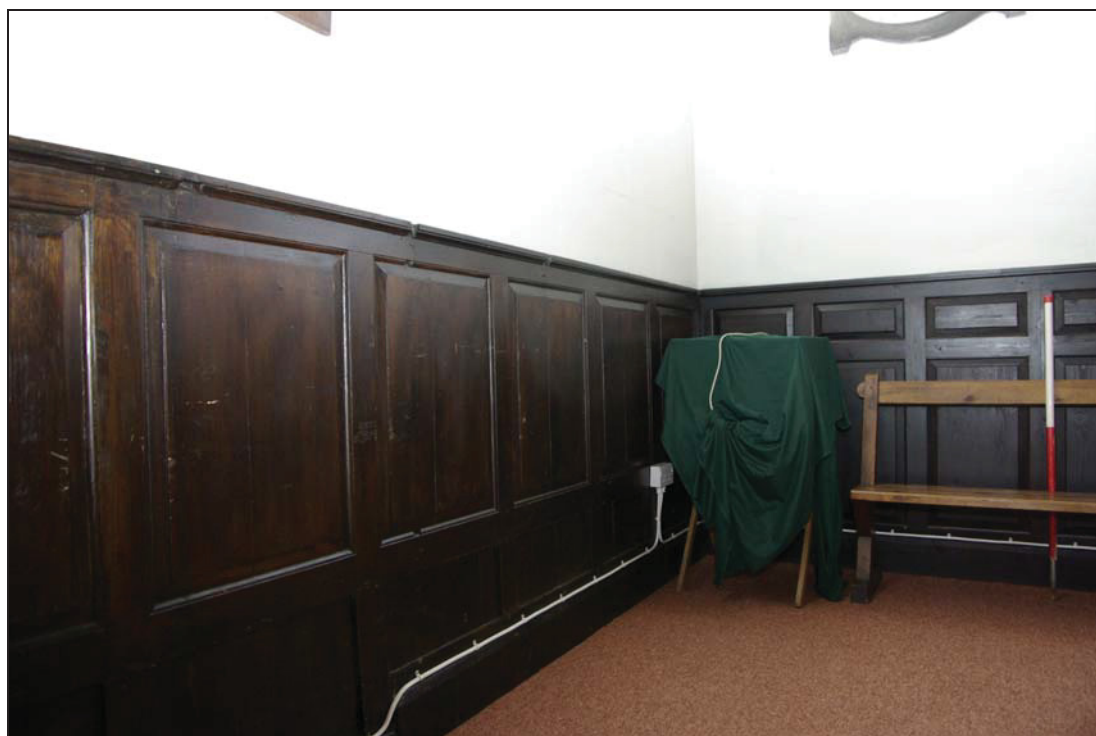
Figure 8. North-west corner of church, with original Georgian wainscoting on left-hand side meeting later Victorian wainscoting lining the northern wall of the nave. Looking north-west.
