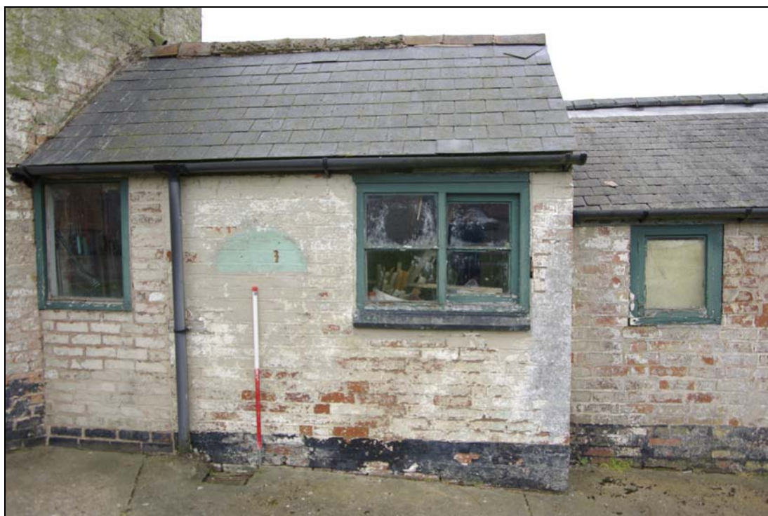
Figure 16. Outbuilding 1, looking east.
