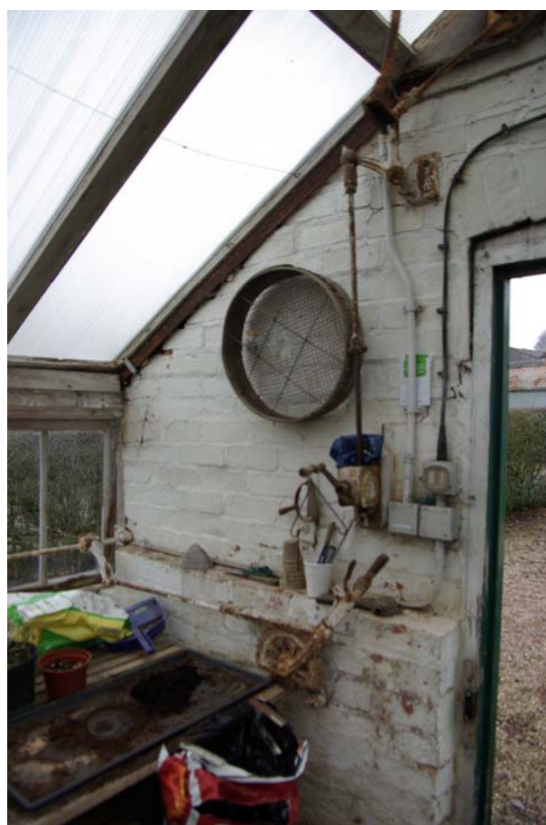
Figure 23. Winding mechanism for opening windows. Looking west.
