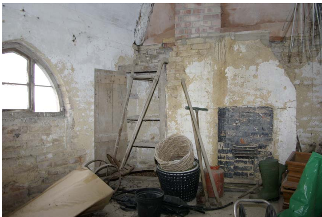
Figure 15. Early fitted cupboard built up against fireplace jamb on upper floor. Looking south.
