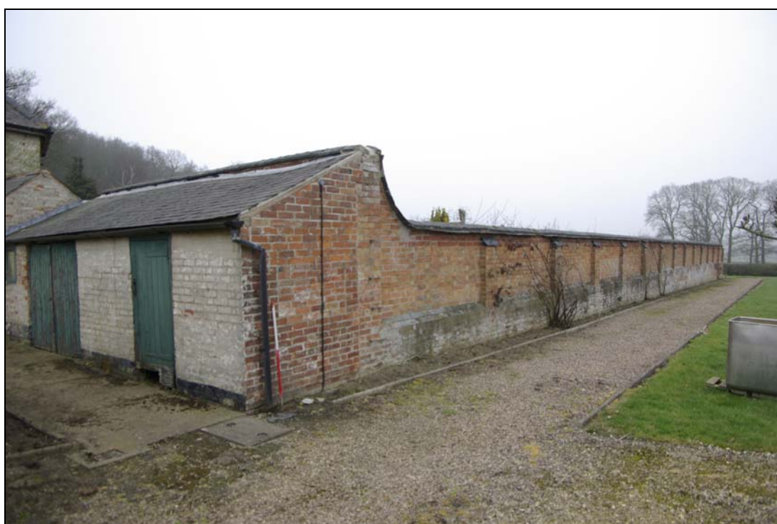
Figure 19. Junction of outbuildings 2 and 3, built-up to garden wall. Looking east.
