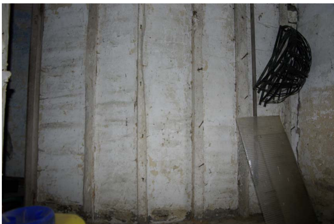
Figure 13. Early stud partition wall to stair hatch. Looking north-east.
