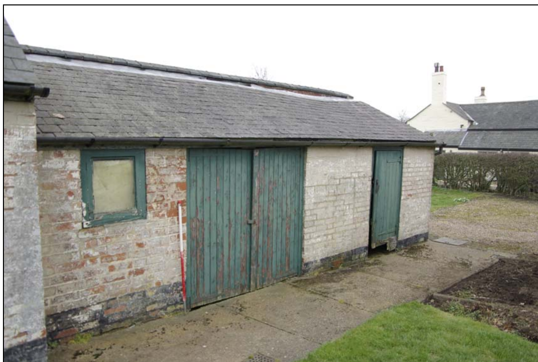
Figure 18. Outbuildings 2 and 3, looking south-east.
