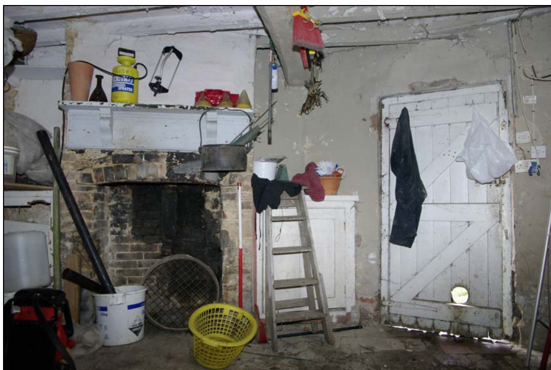
Figure 11. Ground floor fireplace and ledged and braced door. Looking south.
