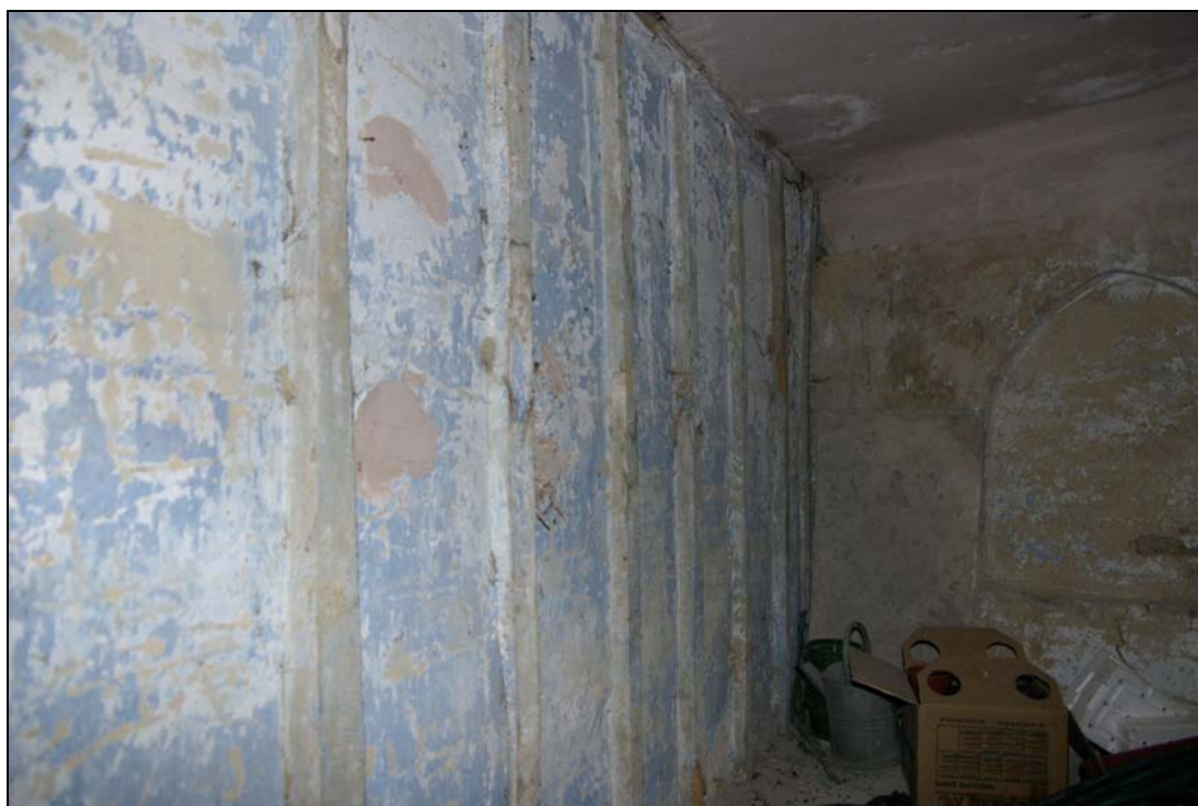
Figure 12. Early stud partition wall, with blind window beyond. Looking south.
