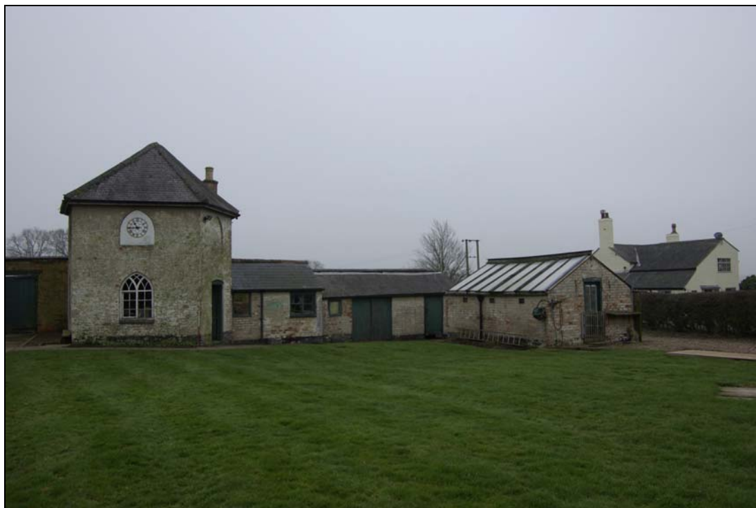
Figure 6. The garden buildings at Billesdon Coplow. Looking east.
