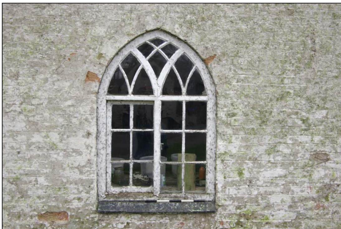
Figure 10. Horizontal sliding sash, with decorative tracery above. Looking south-east.
