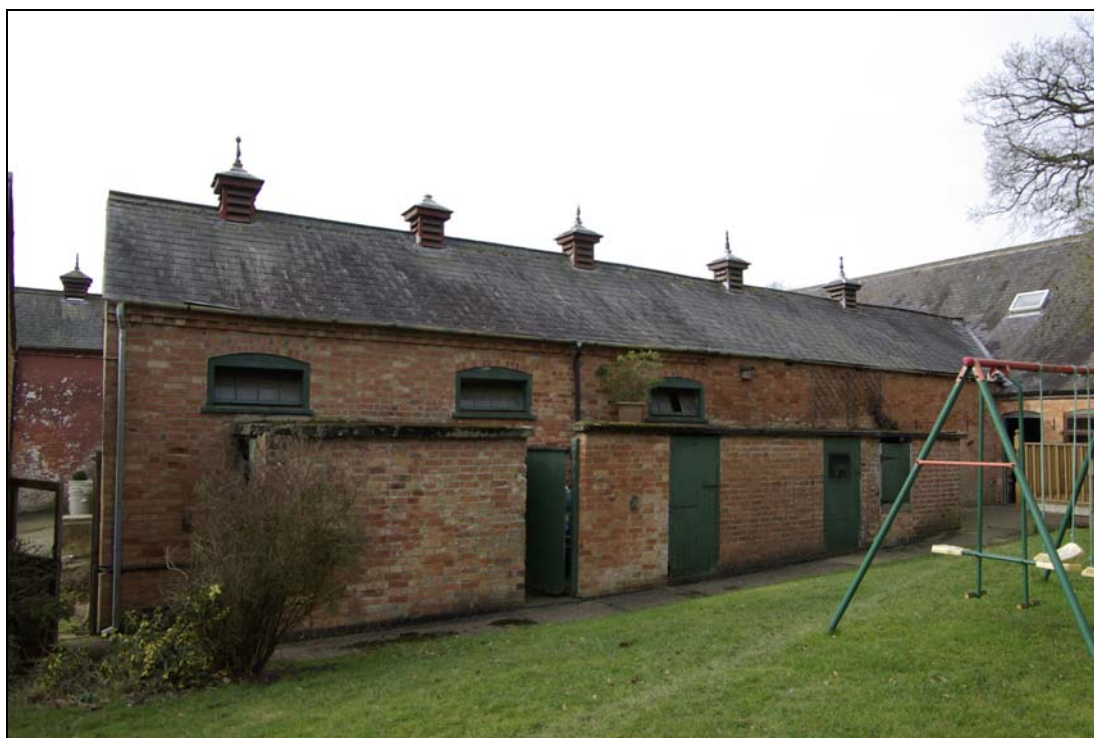
Figure 10. Rear elevation of north-eastern stable range, looking west.
