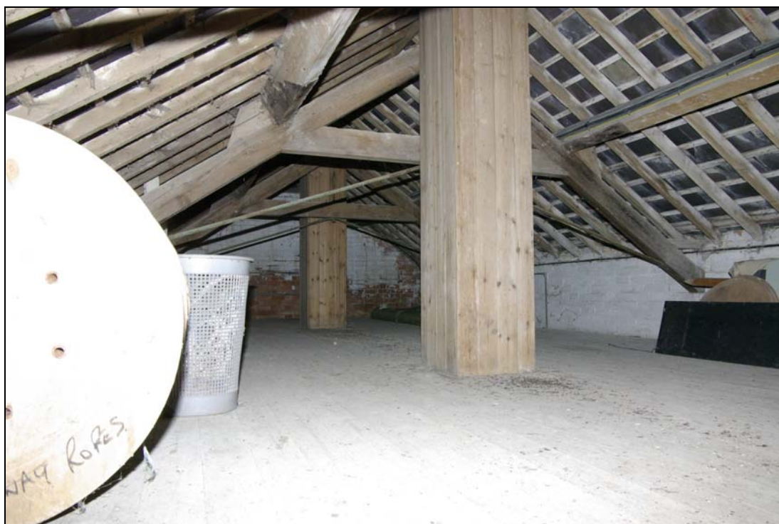
Figure 17. Upper hay loft, with timber ventilation shafts. Looking north-west.
