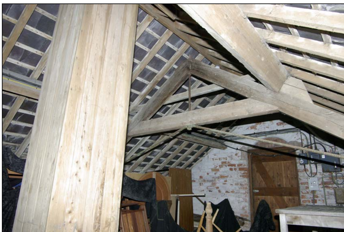
Figure 18. Principal roof truss with king-bolt, in hayloft looking east.
