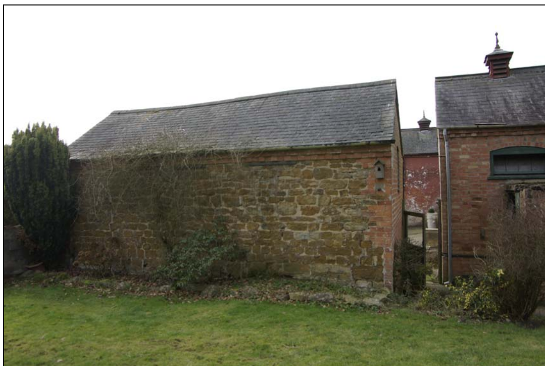
Figure 13. Iron-stone wall to rear of apple store. Looking south-west.
