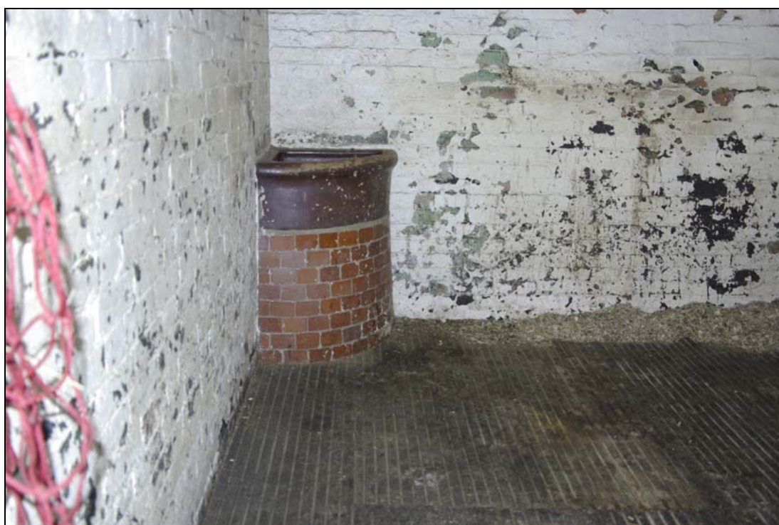
Figure 14. Glazed brick and ceramic feeding trough, stamped Oates and Green Ltd, Halifax. Looking north-east.
