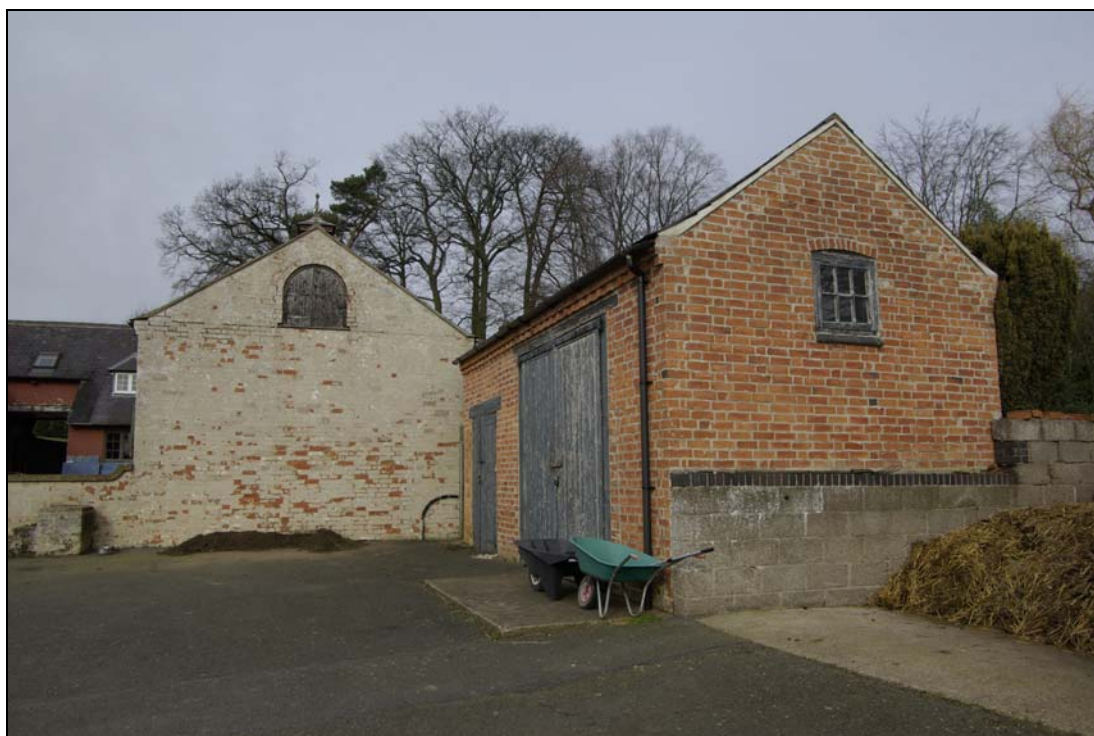
Figure 12. Apple store, looking north.
