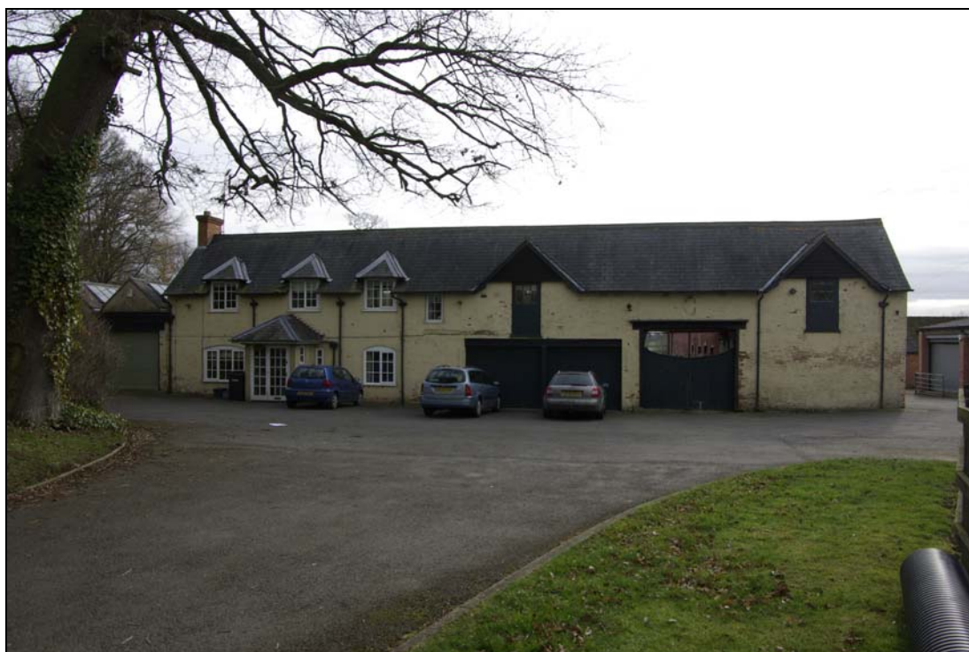
Figure 5. Stable- block, frontage range, looking south-east.
