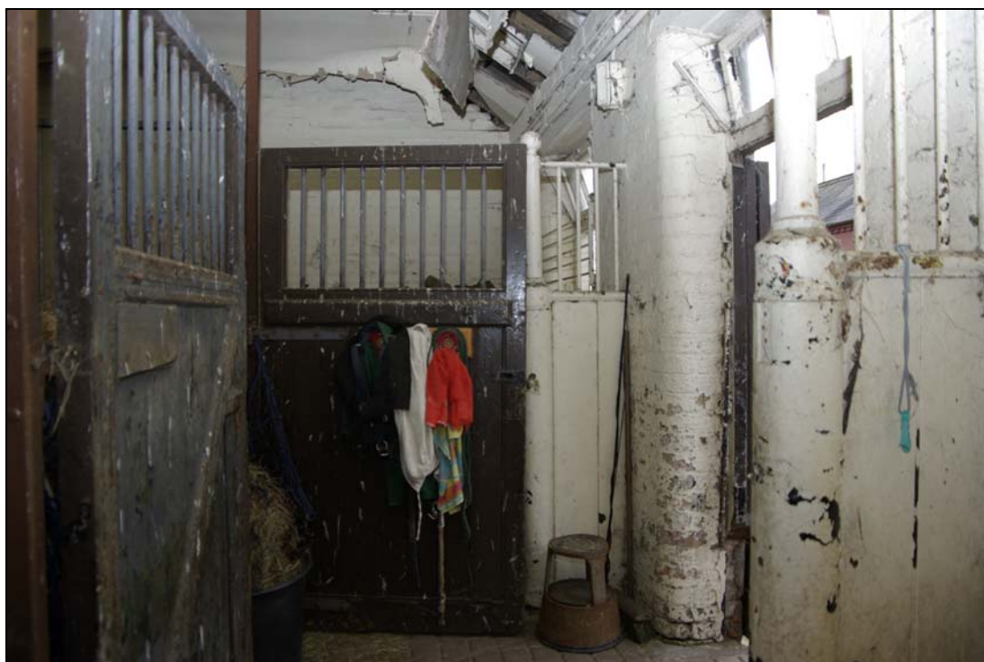
Figure 15. Ledged and braced door to loose-box, with cast-iron post. Looking south-east.
