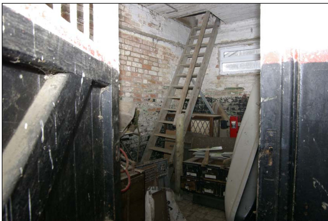
Figure 16. Stair ladder to upper hay-loft. Looking south.
