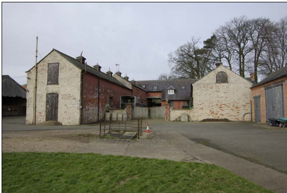
Figure 11. Stables, looking north-west towards livery yard.
