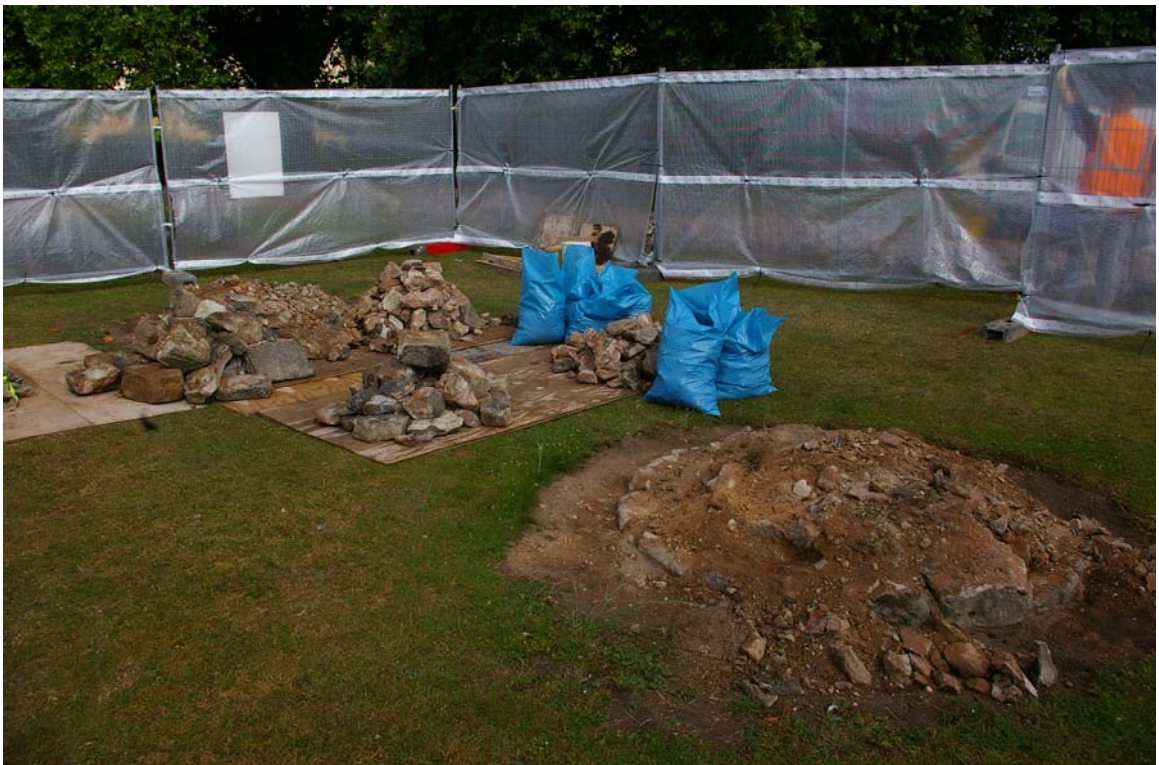
Figure 6. Working shot during dismantling of piers 1 and 2. Looking west
