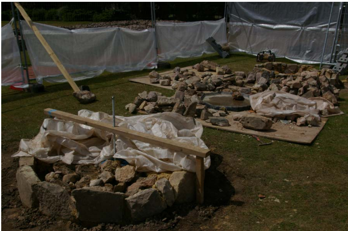
Figure 10. Reconstruction of piers 1 and 2, looking west.
