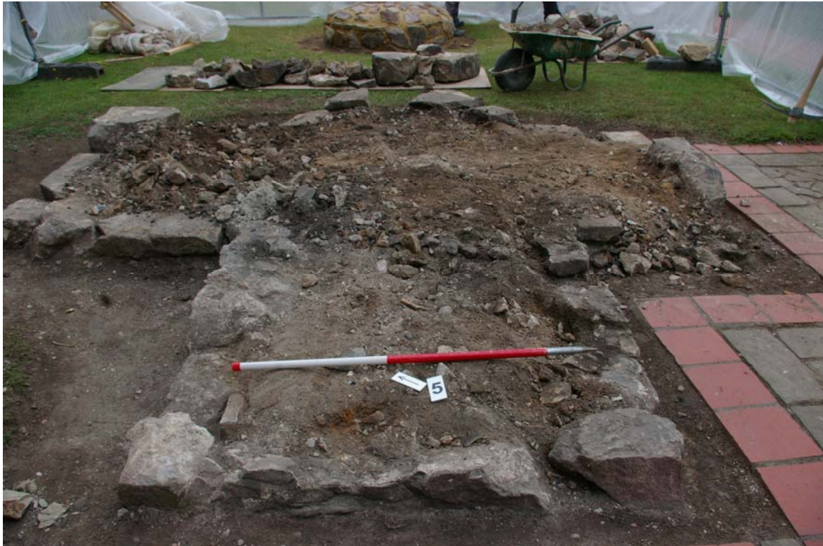
Figure 9. Dismantling of pier 5, at base of tower. Looking east.
