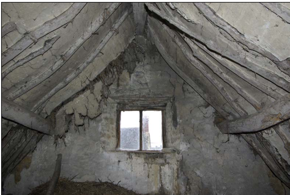
Plate 25. 2nd floor attic room, looking south.
