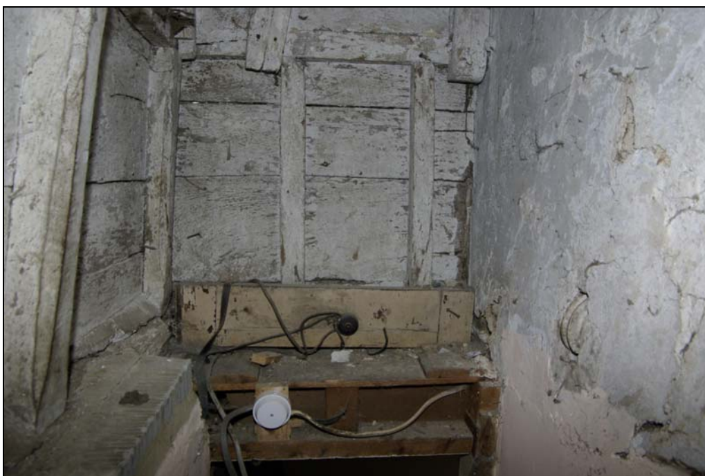
Plate 23. As above, access hatch in floor, with pulley wheel for hoist located on right-hand side. Looking west.
