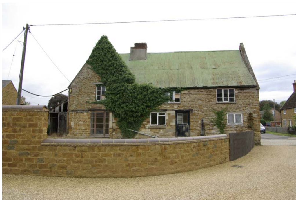
Plate 3. Rear elevation, looking east.
