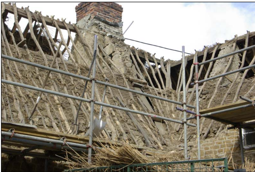
Plate 10. Detail of above, showing rafters pegged into backs of purlins.
