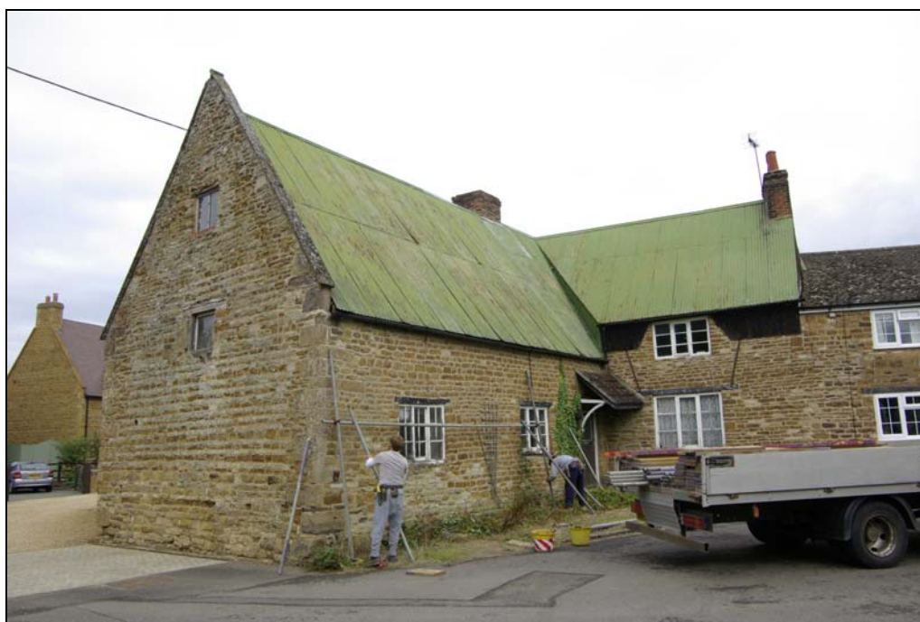
Plate 2. Westhorpe farmhouse, frontage elevation, looking north-west.
