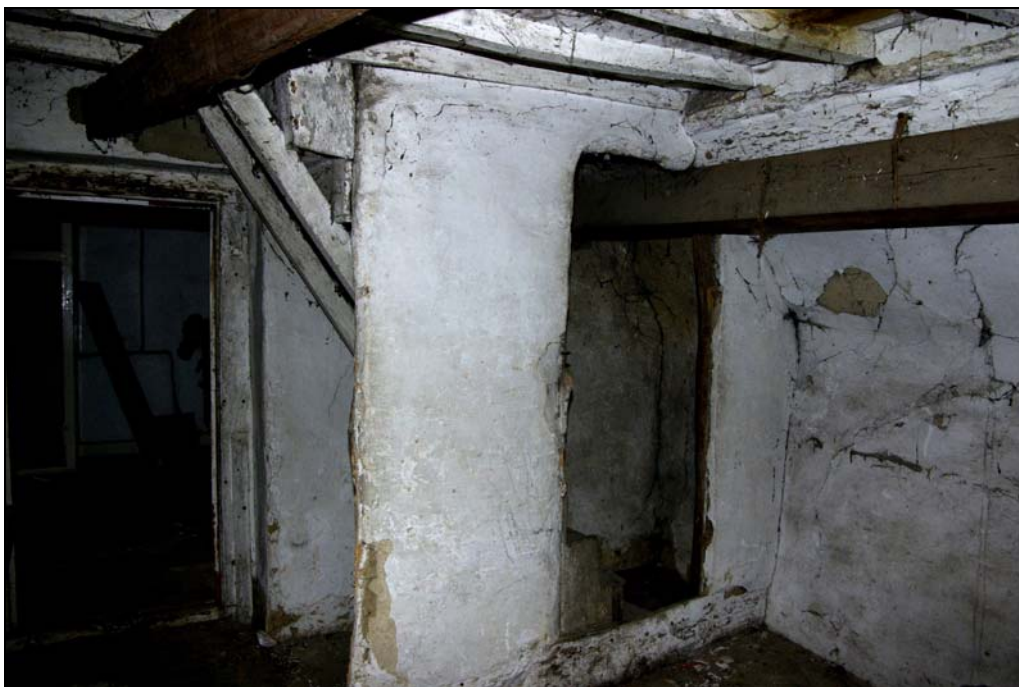
Plate 24. As 22, boxed-in ladder stair to 2nd floor attic room. Looking north-east.
