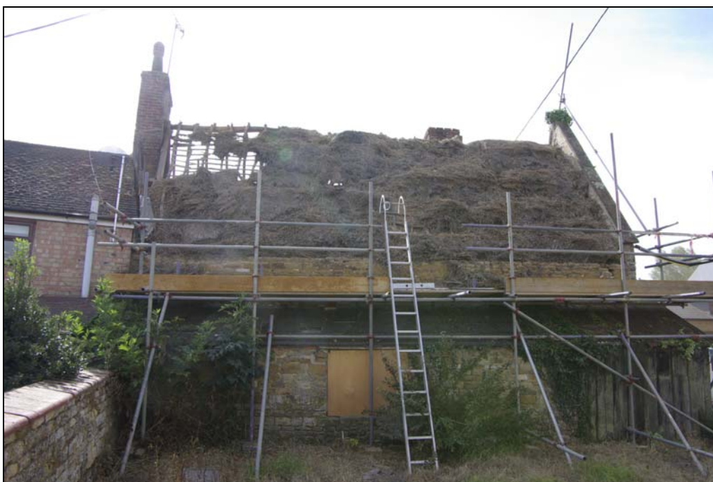
Plate 8. Looking south, during removal of thatch.
