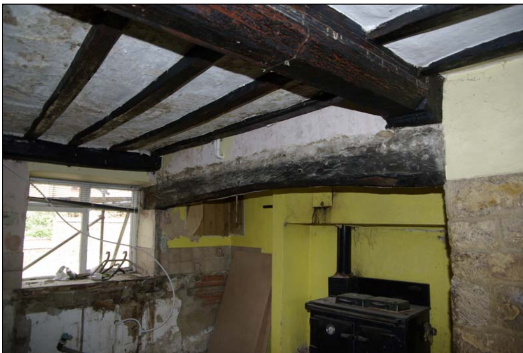
Plate 11. Ground floor living kitchen.
