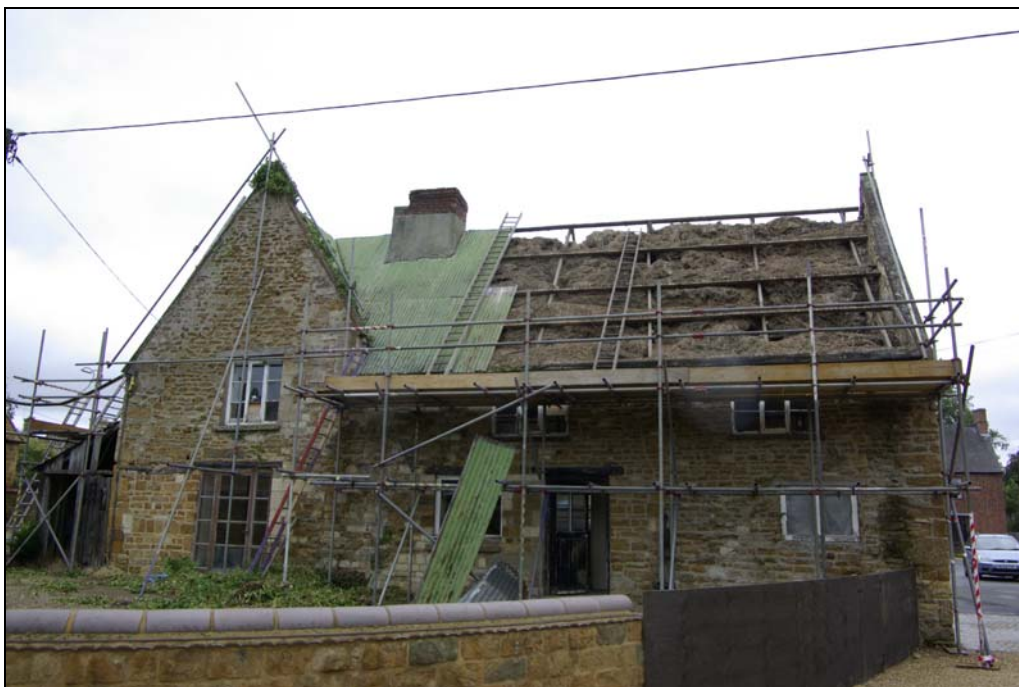
Plate 7. Rear, during removal of tin cover.
