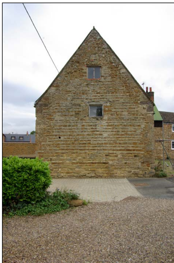
Plate 5. Southern gable end, looking north.
