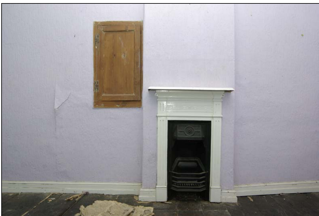
Plate 21. First floor chamber, with 19th century cast-iron fireplace and fitted cupboard with 18th century H-hinges. Looking south.
