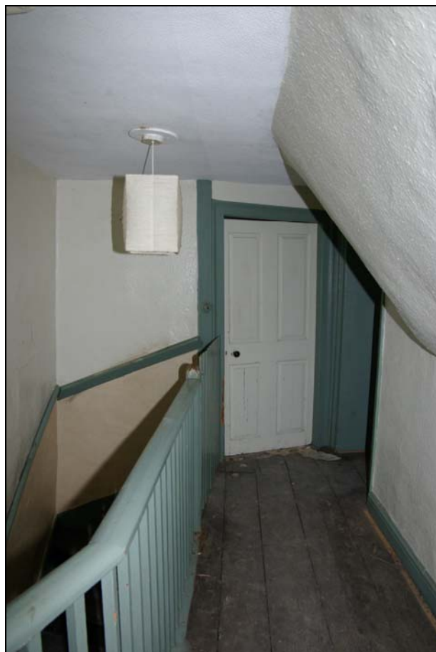
Plate 18. First floor landing, looking north.
