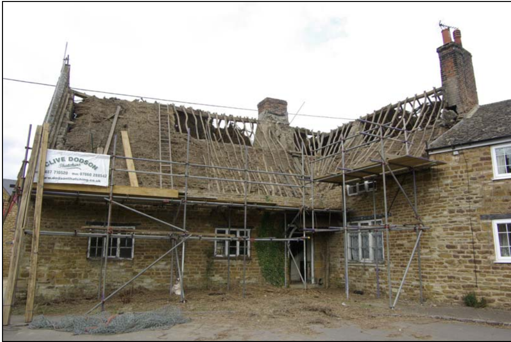
Plate 9. Exposed rafters, following removal of thatch.
