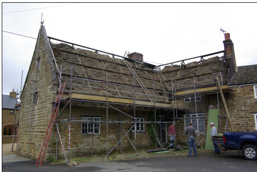
Plate 6. Frontage, following removal of tin cover.
