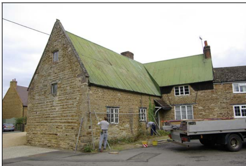
Plate 1. Westhorpe Farmhouse, front elevation, looking north-west.
