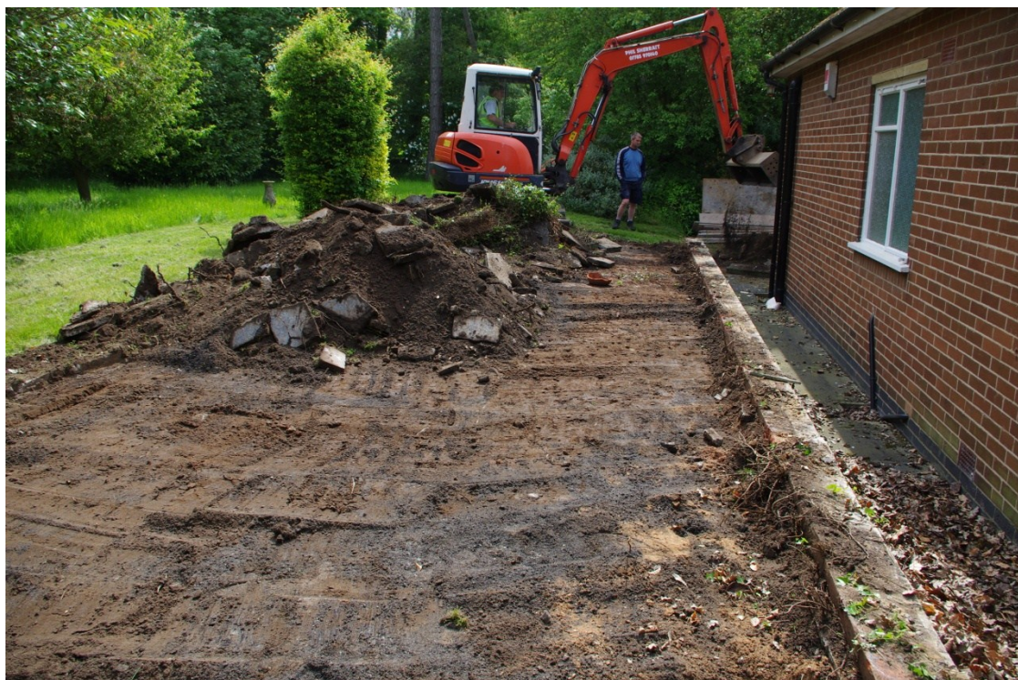
Figure 5 Removal of the patio, north-eastern area. Looking east
