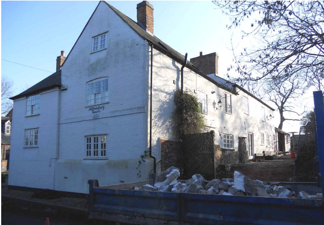
Figure 4. 31 Swan Street. Looking south-east
