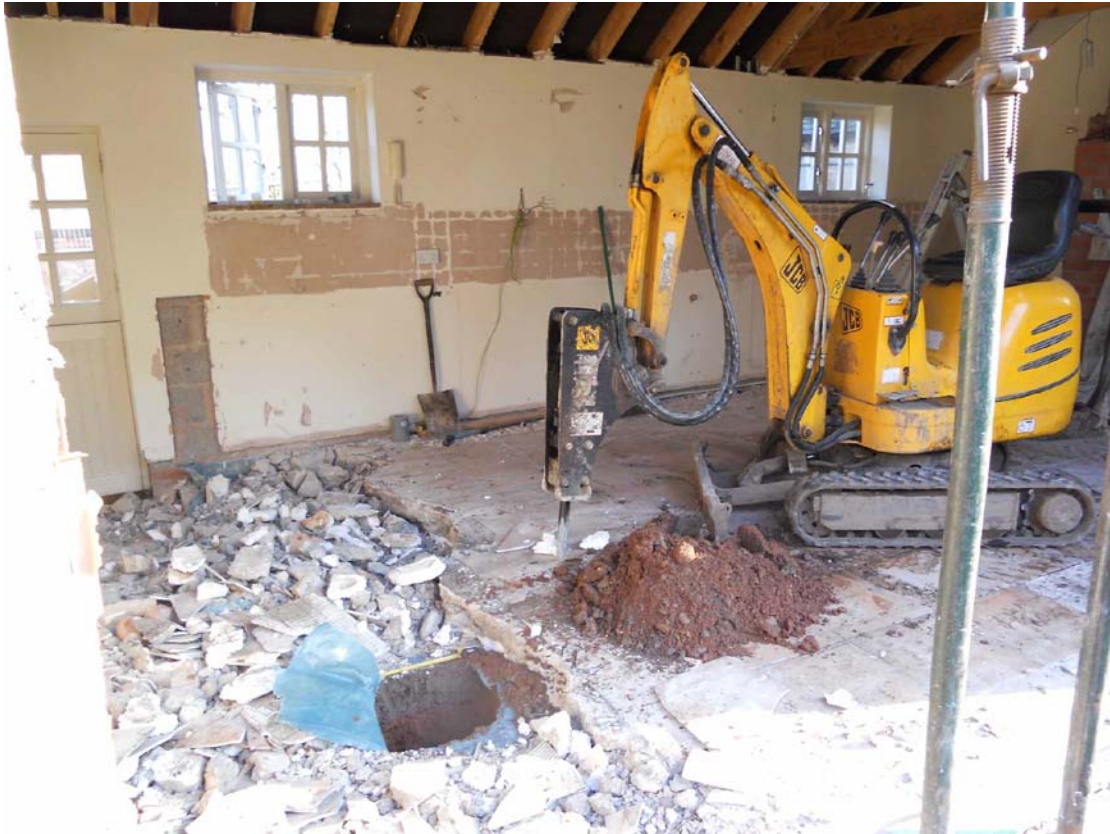
Figure 6. Modern floor being removed after soft strip. Looking south-east
