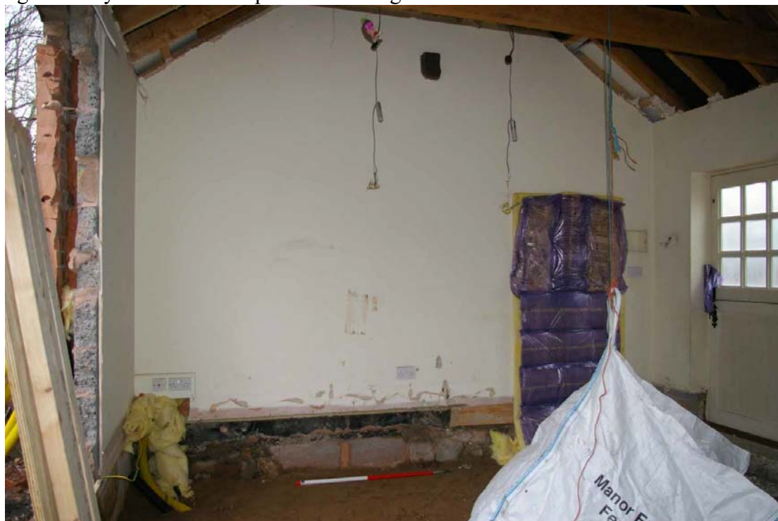
Figure 8. Blocked doorway Note projecting beam in gable. Looking north. 1m scale
