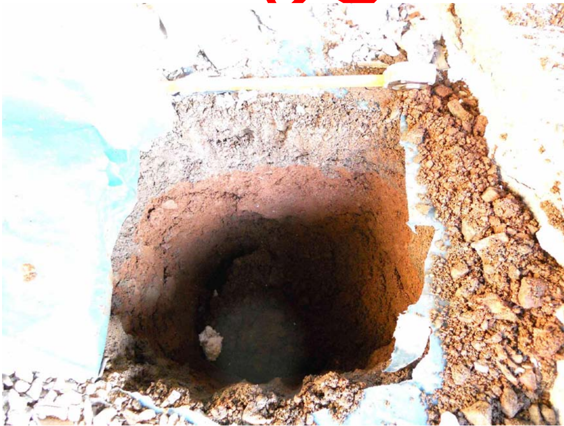
Figure 7. Sample excavation to assess depth of floor.
