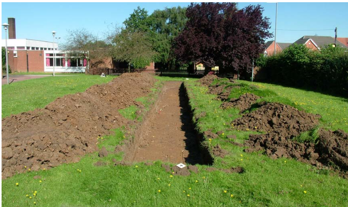
Plate 2: Trench after excavation, looking north-west
