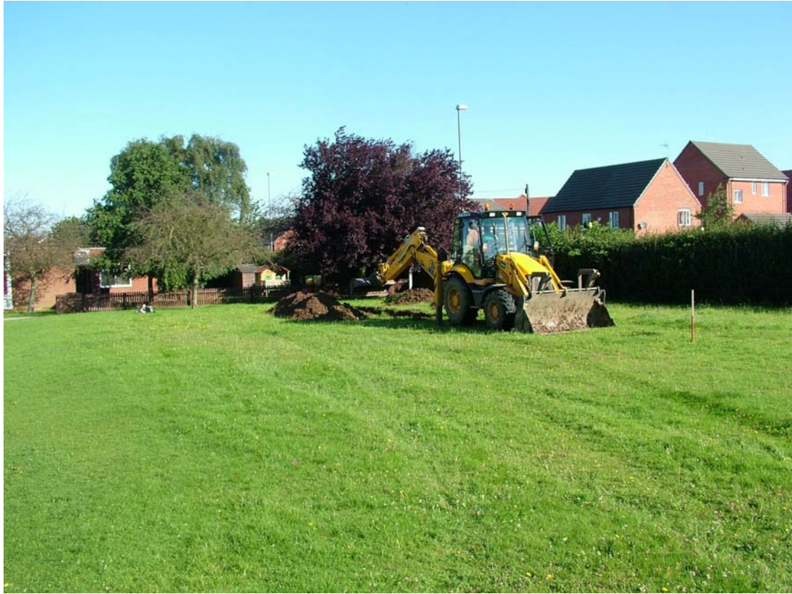
Plate 1: Work in progress, looking north
