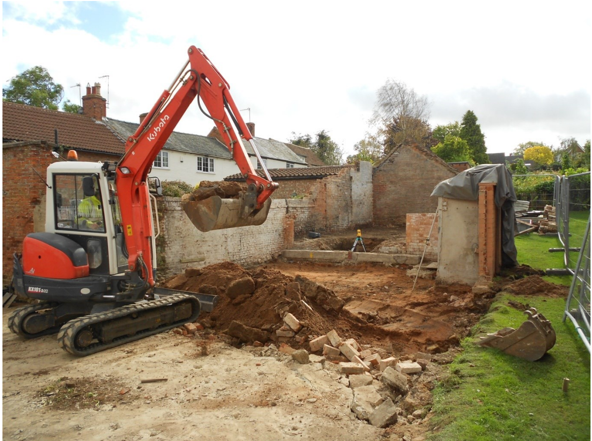
Figure 4: Concrete / hardcore being removed
