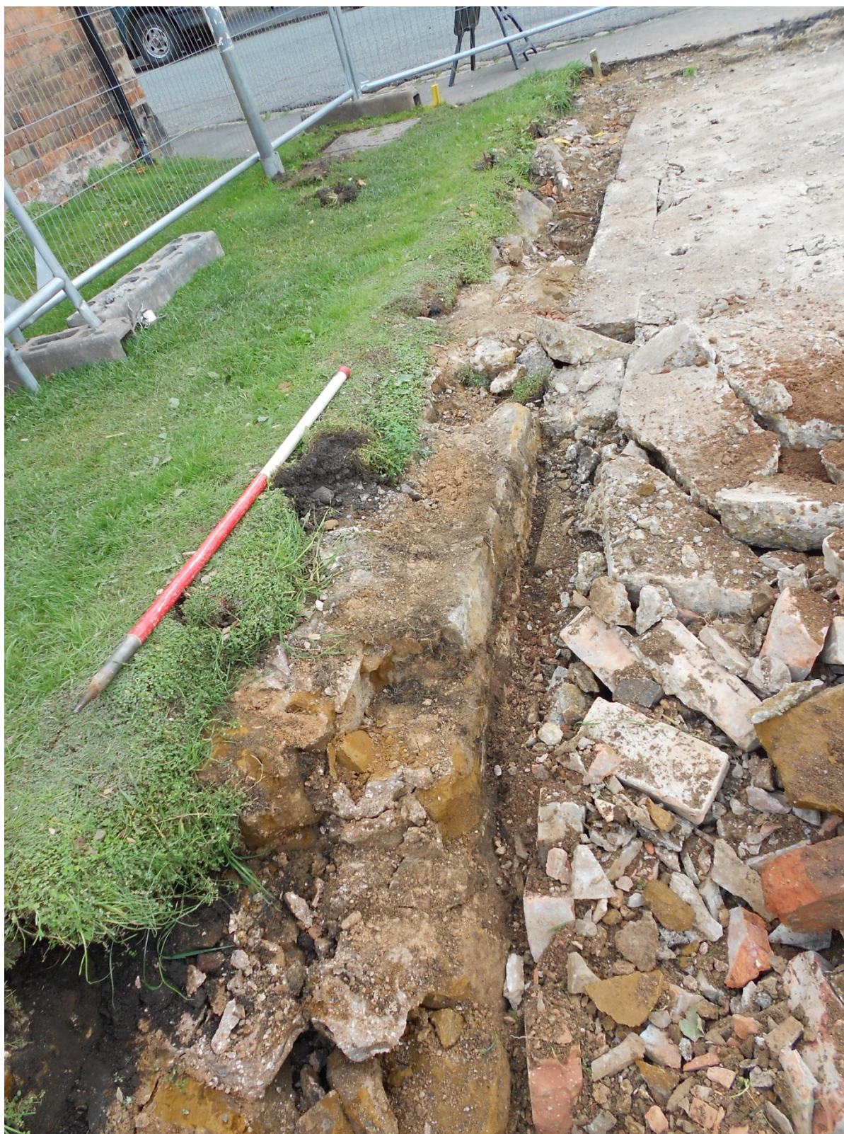
Figure 10: Stone footings, 1m scale, looking north towards street-frontage
