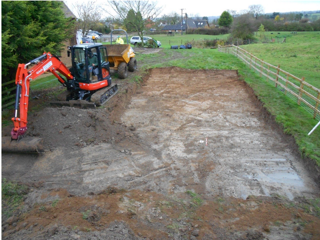
Figure 5: View of excavation in progress, looking east, 1/2 metre scale.
