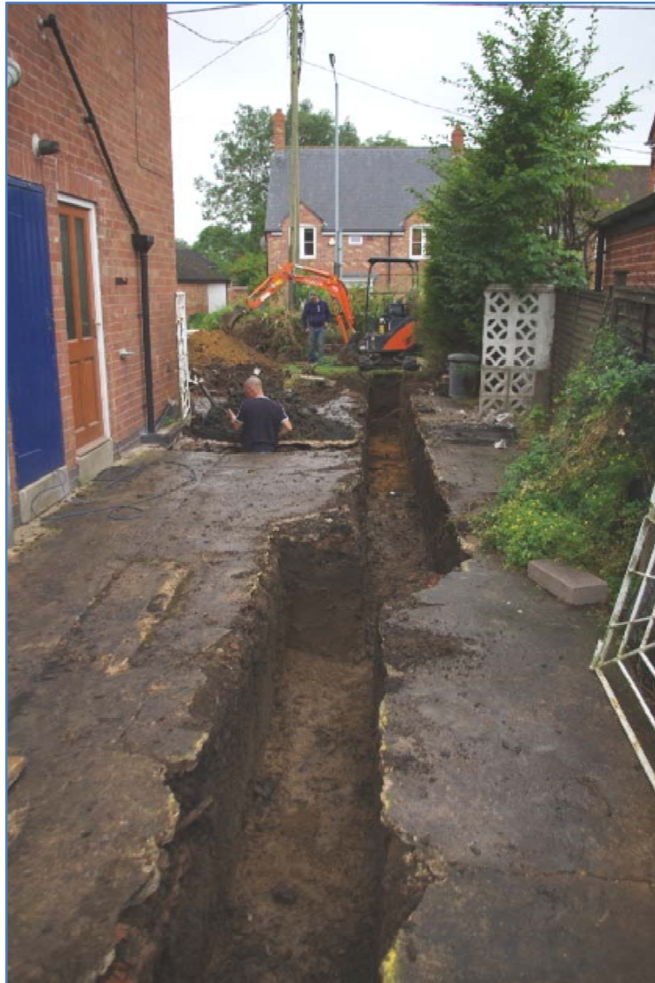
Figure 6: Footing dug through concrete apron. Looking SSW.
