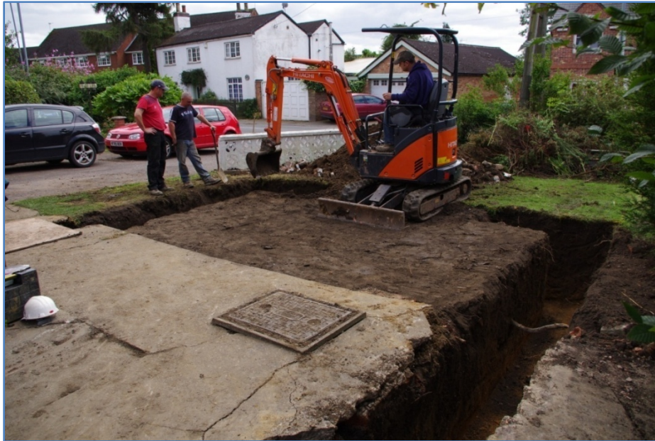
Figure 4: The proposed garage area in front of the property. Looking south.
