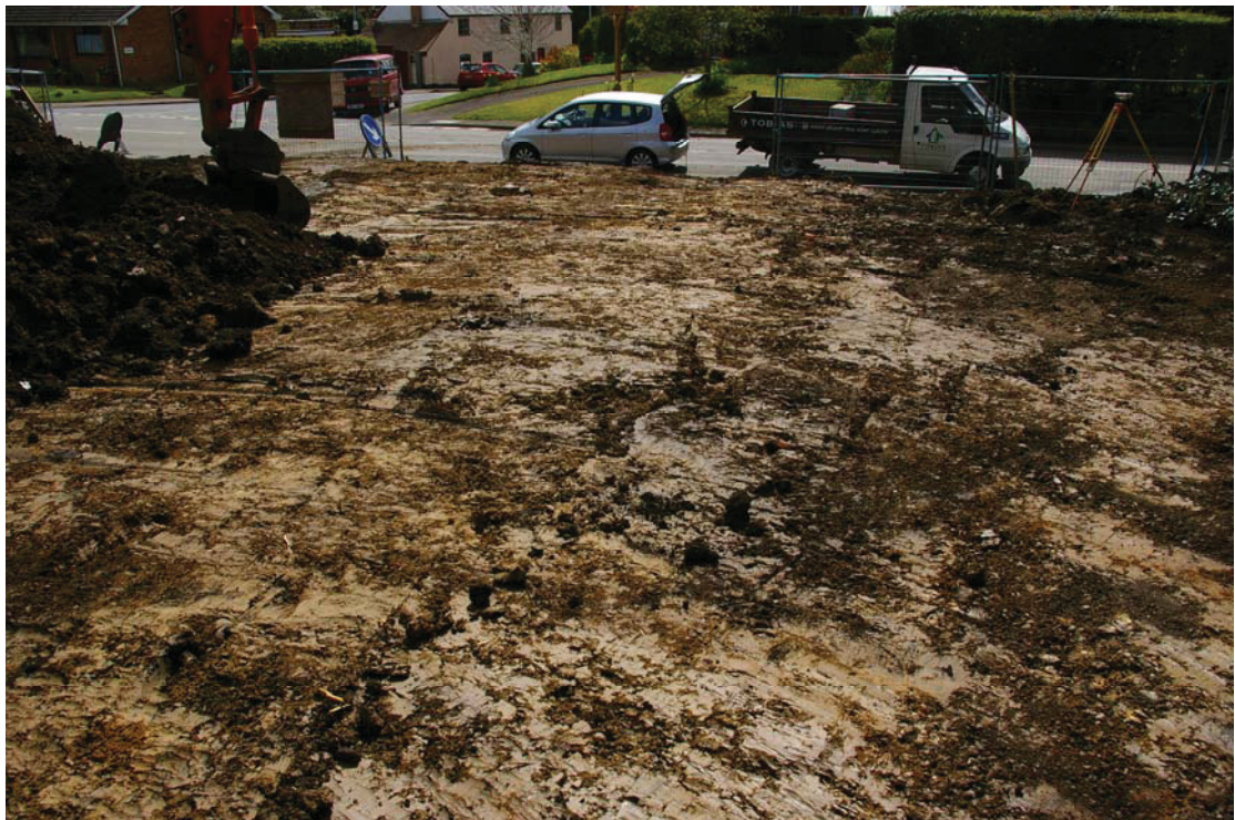
Plate 8: Street frontage area stripped, looking south-east
