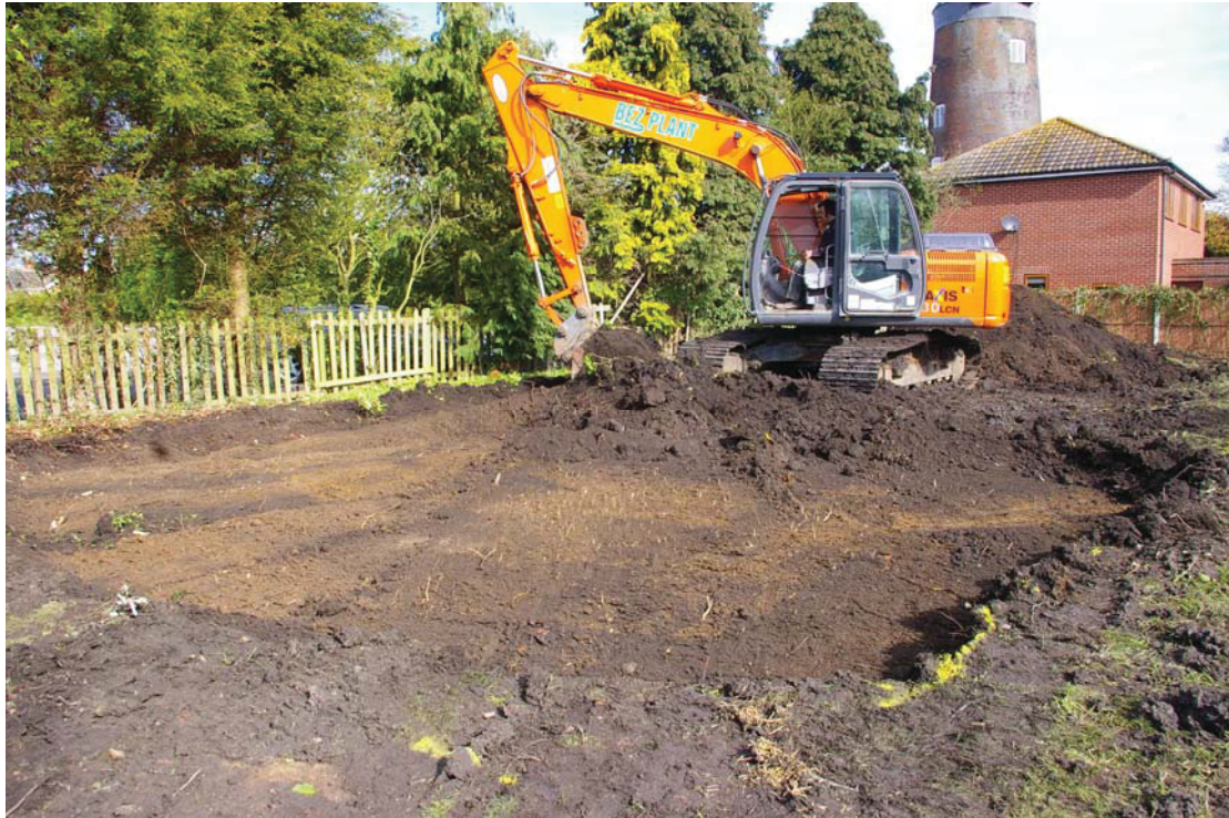
Plate 3: Work in progress on garden area. Looking north-west
