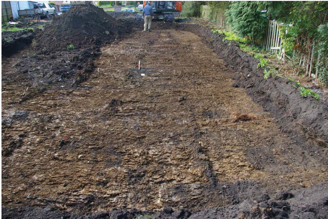
Plate 5: Western part of garden area stripped, looking south
