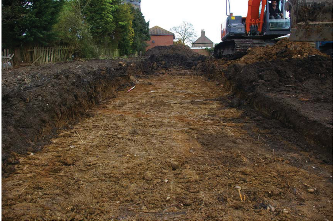
Plate 7: Finished initial strip at street frontage, looking north
