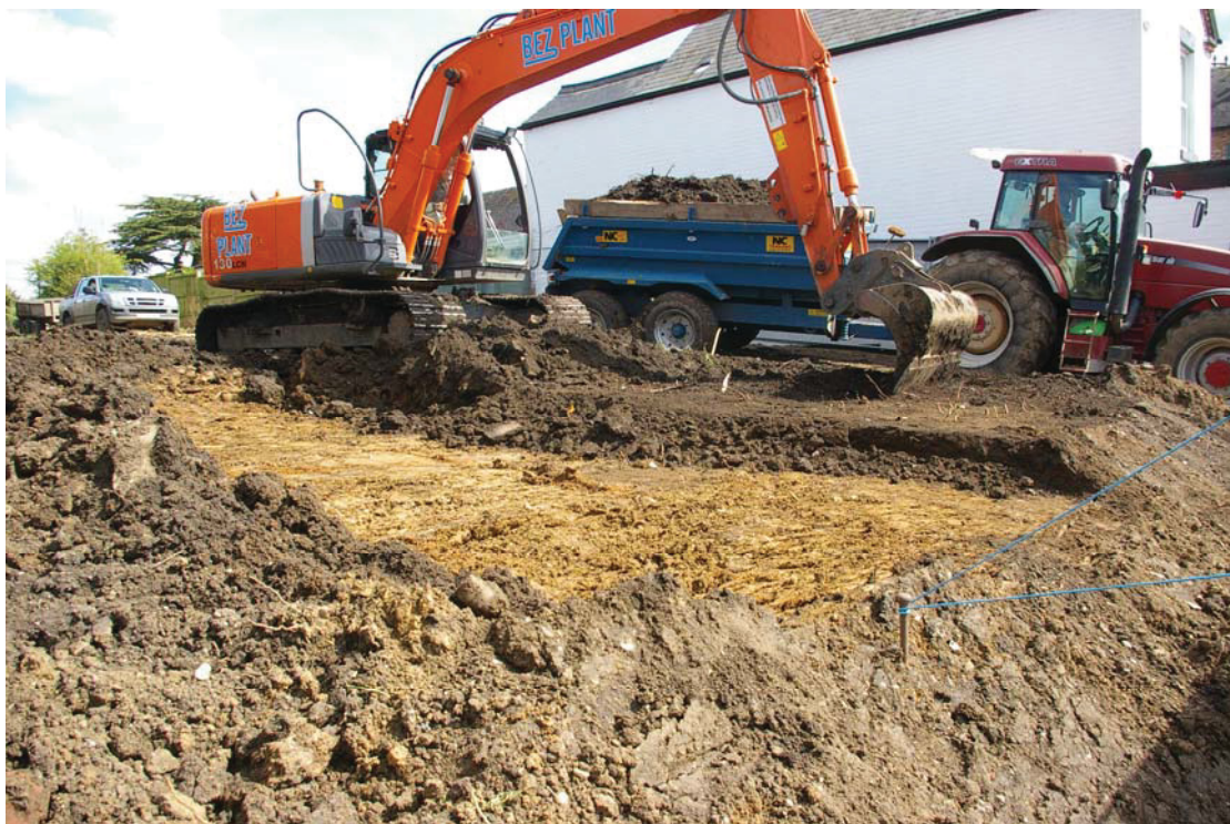
Plate 6: Work in progress at street frontage, looking north-east
