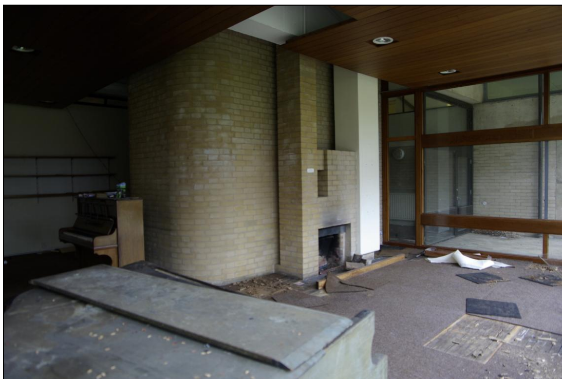
Figure 37. Ground floor common room, looking north-east.
