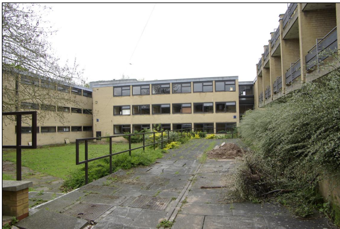
Figure 12. Southern courtyard, looking west towards Block A.
