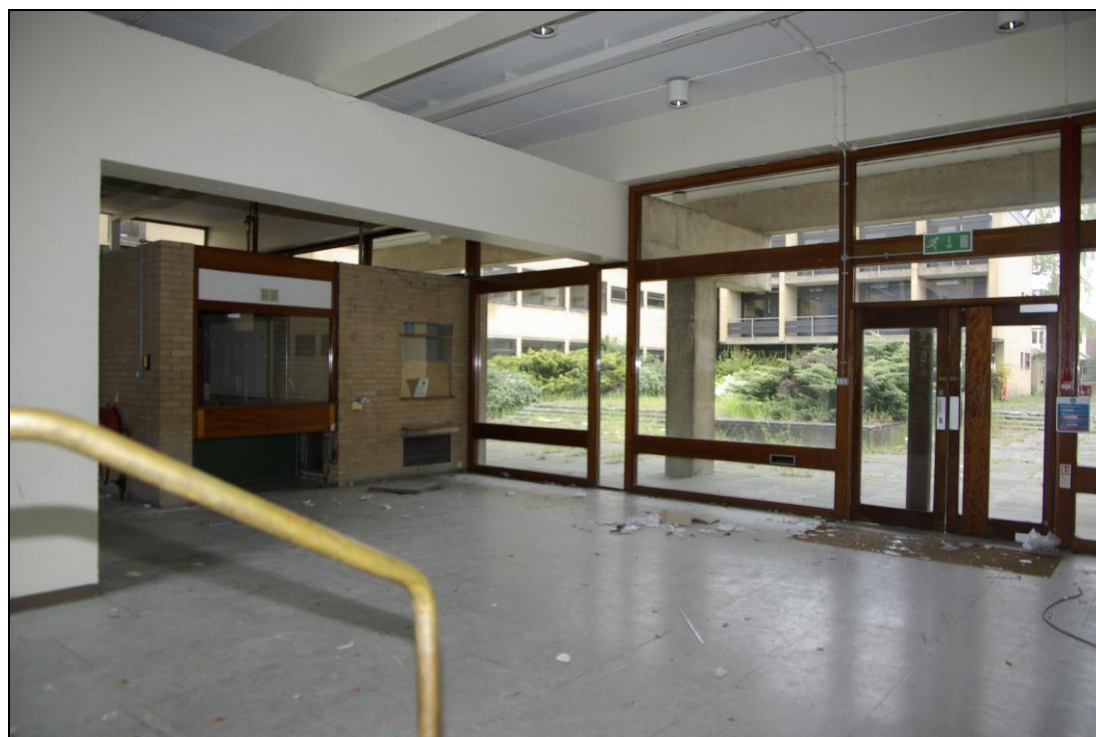
Figure 28. Block D, foyer and reception, looking north-west.
