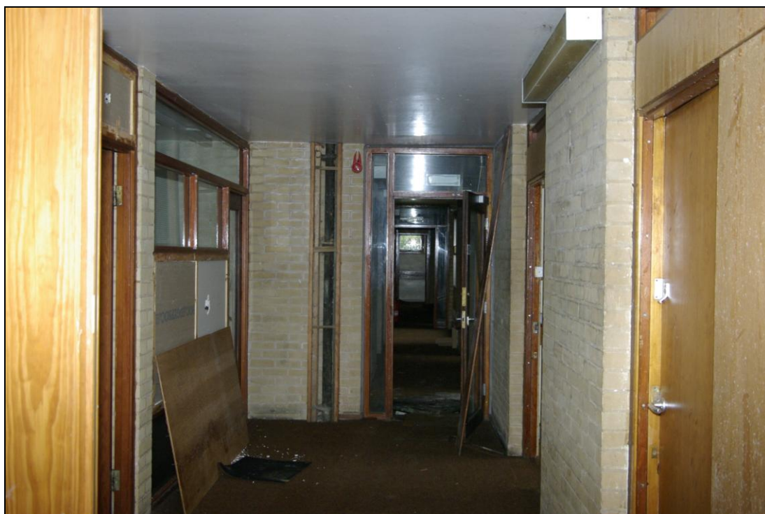
Figure 23. Central corridor, Block A, looking north.
