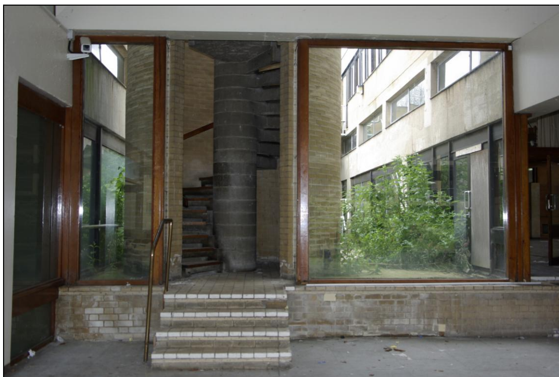
Figure 30. As above, looking south towards stairwell.
