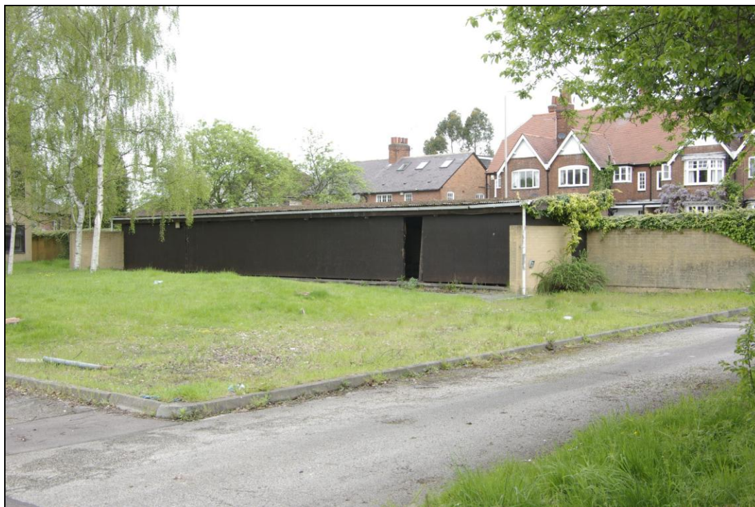
Figure 5. Bike shed, looking north-west.
