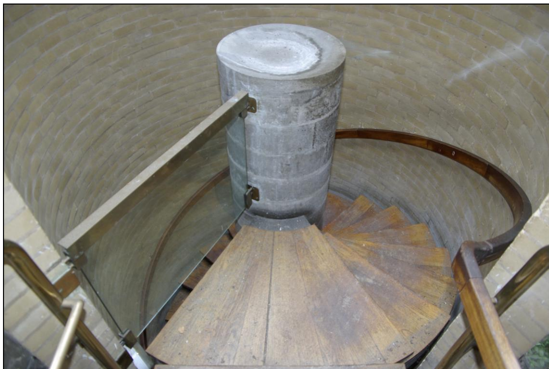
Figure 31. Top of staircase, Block D first floor, looking south.
