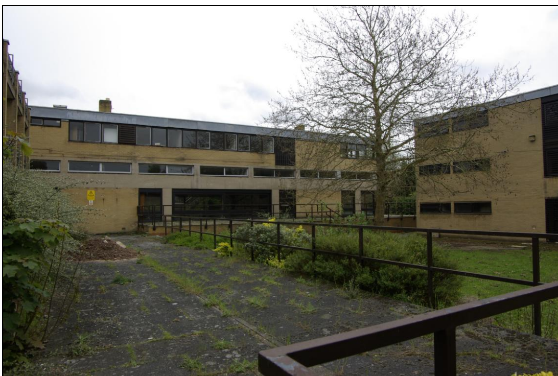
Figure 14. As above, looking south-east towards Block D.
