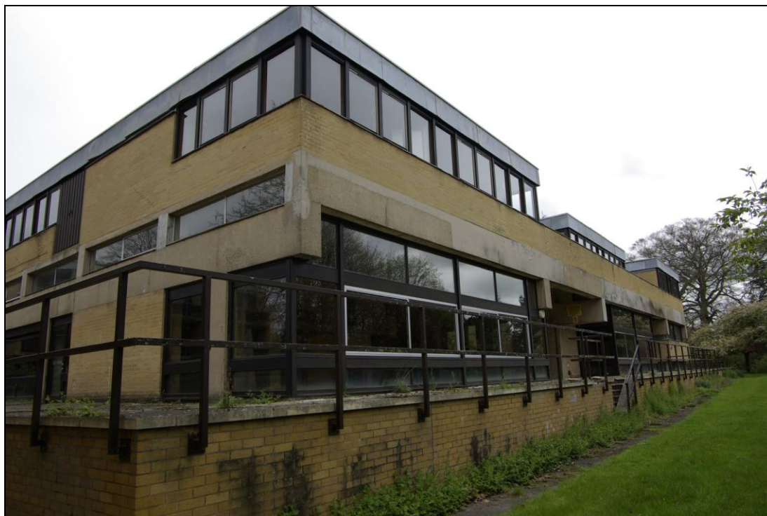
Figure 17. Block D, looking north-east.
