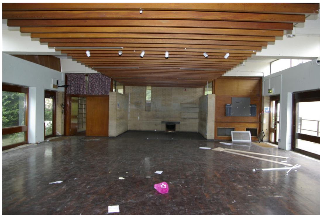
Figure 35. Bar, looking south.
