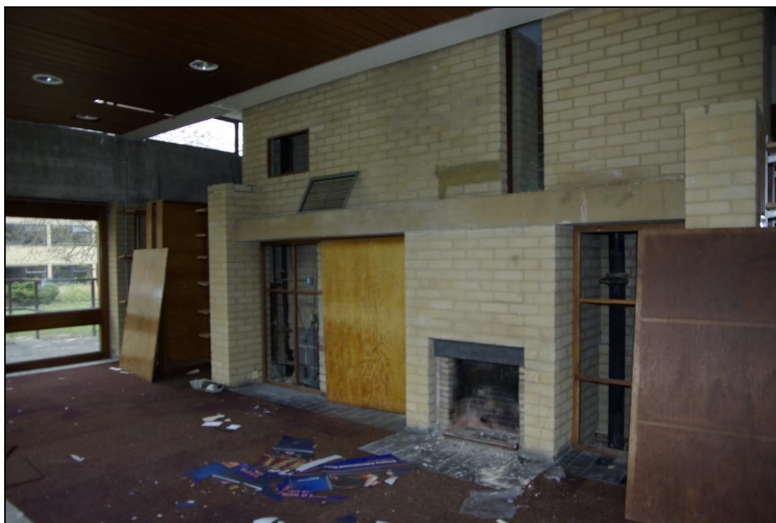
Figure 36. Heated library, looking north-west.
