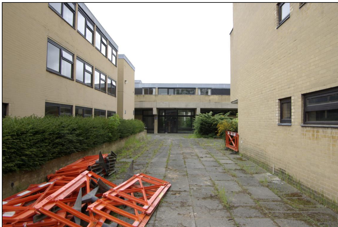
Figure 7. Corridor between blocks B and C, looking south towards Block D.
