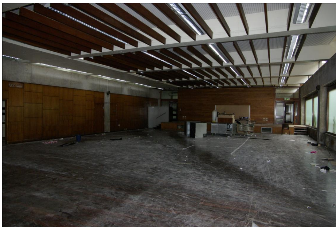
Figure 32. Refectory, looking south-east.
