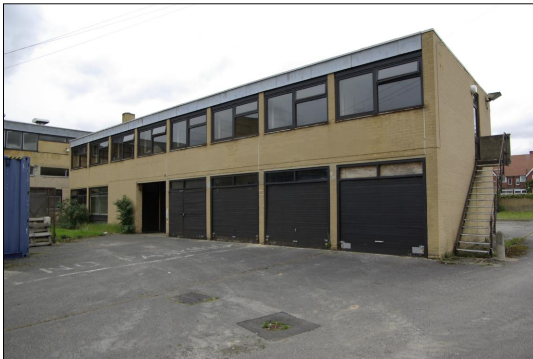
Figure 21. Block E, looking north-west.
