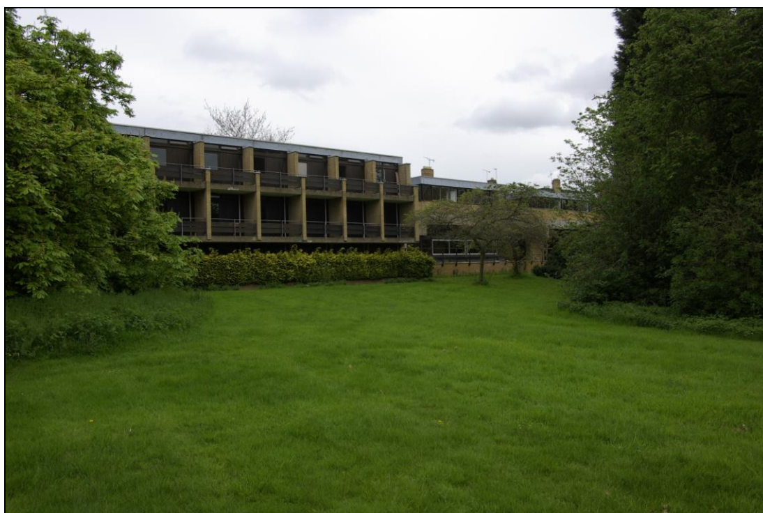
Figure 16. Blocks A and D, looking north-east.
