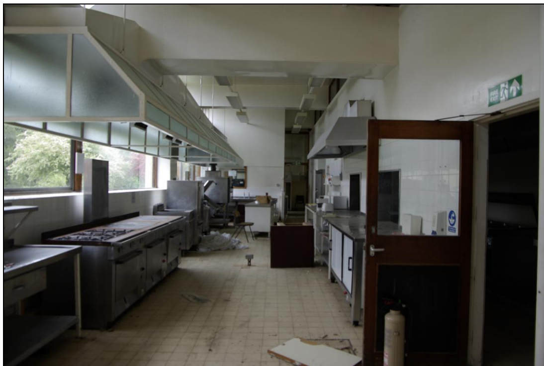
Figure 33. Kitchen, looking south.
