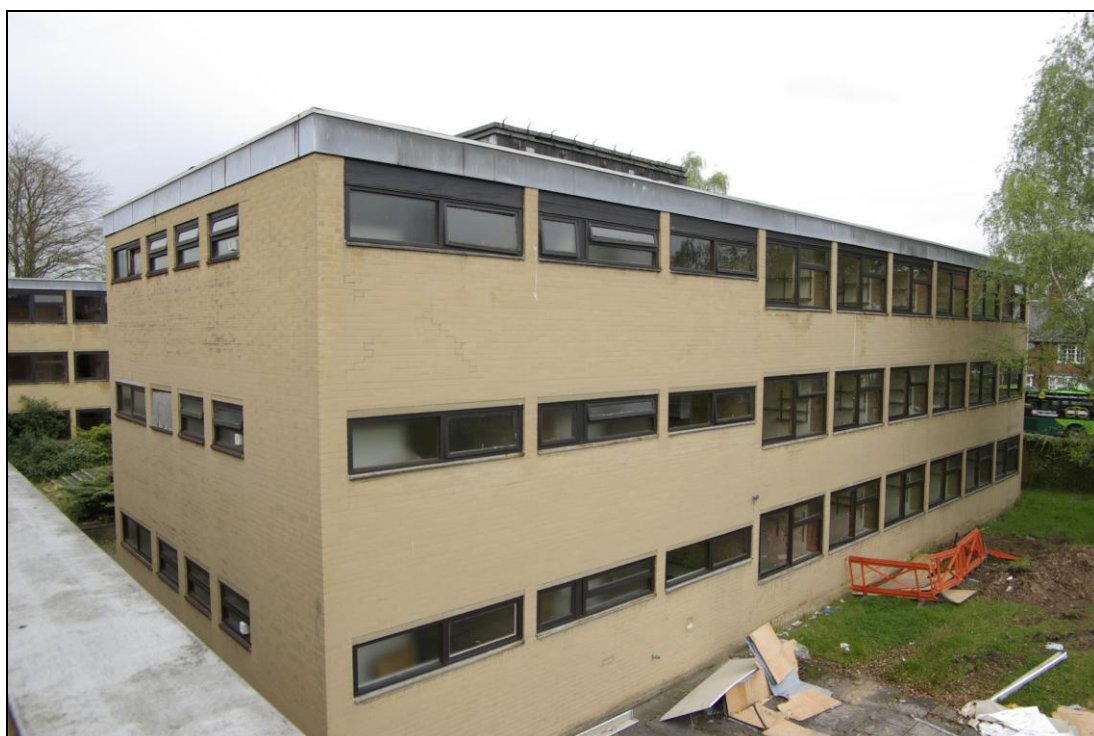
Figure 10. Block C, looking north-west.
