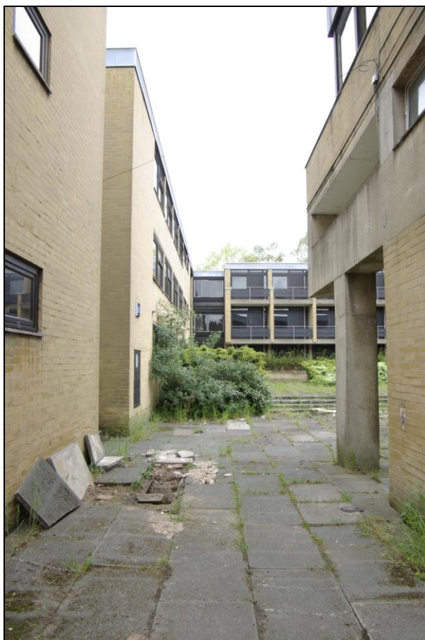
Figure 11. Corridor between Blocks B and D, looking north towards Block B.
