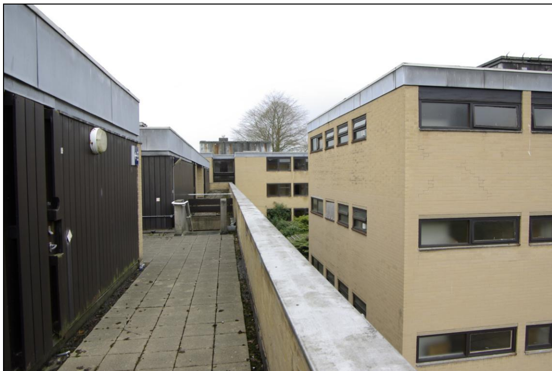
Figure 9. Block D, first floor walkway, looking west.
