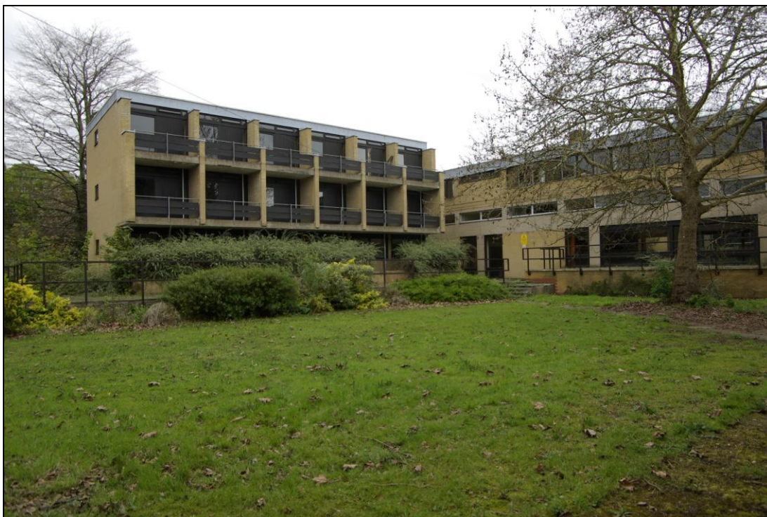
Figure 13. As above, looking north-east towards Block B.
