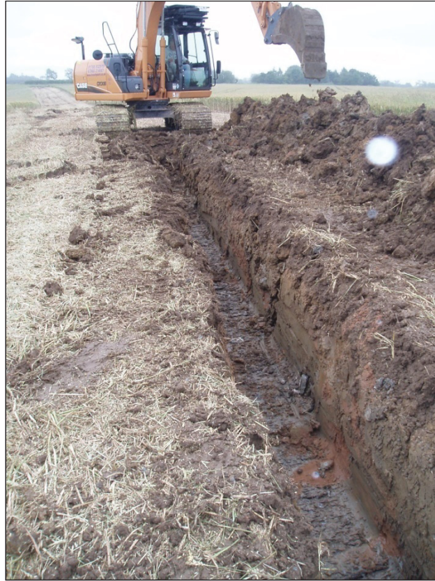
Figure 8: Excavation of cable trench, looking east.
