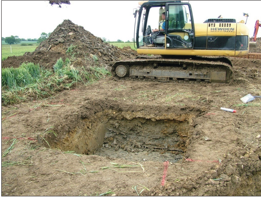
Figure 6: Excavation of substation footprint, looking north.
