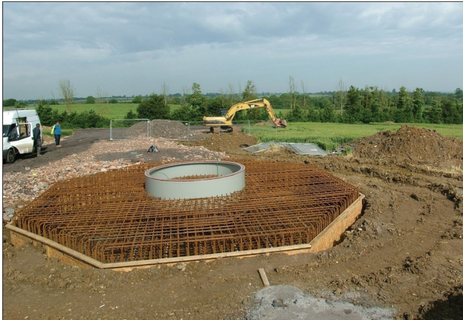
Figure 5: Turbine base, looking north towards site of substation.
