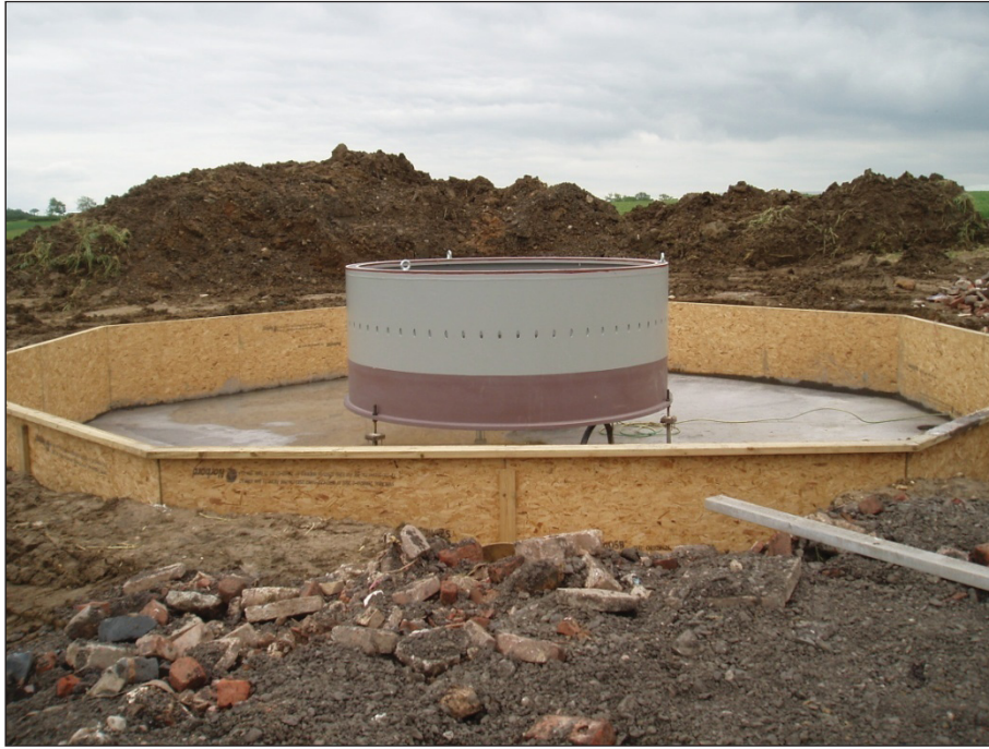
Figure 4: Turbine base, looking north.
