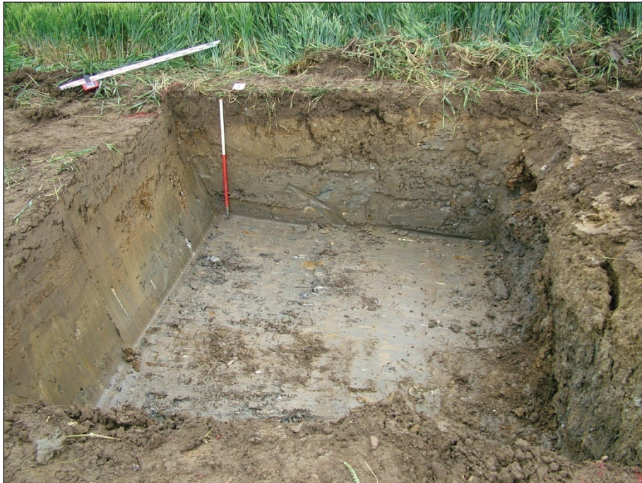
Figure 7: Substation footprint, looking north.
