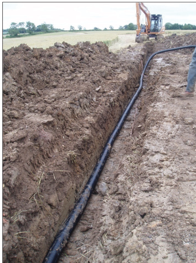
Figure 9: Laying of cable within trench, looking east.
