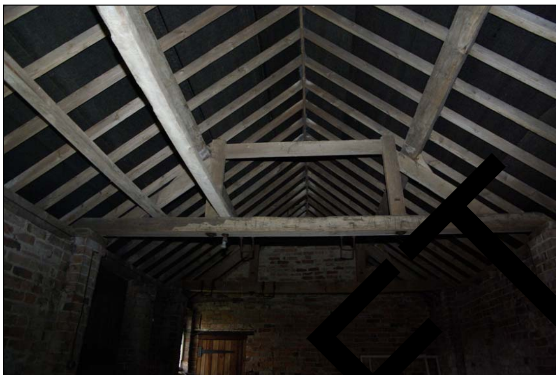
Figure 23. Queen-post roof structure in cow-shed looking north-east.
