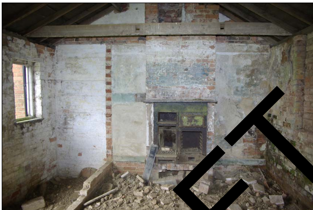
Figure 19. Cast-iron kitchen range and partially demolished single-skin brick wall, possible relics of earlier farmhouse. Looking east.
