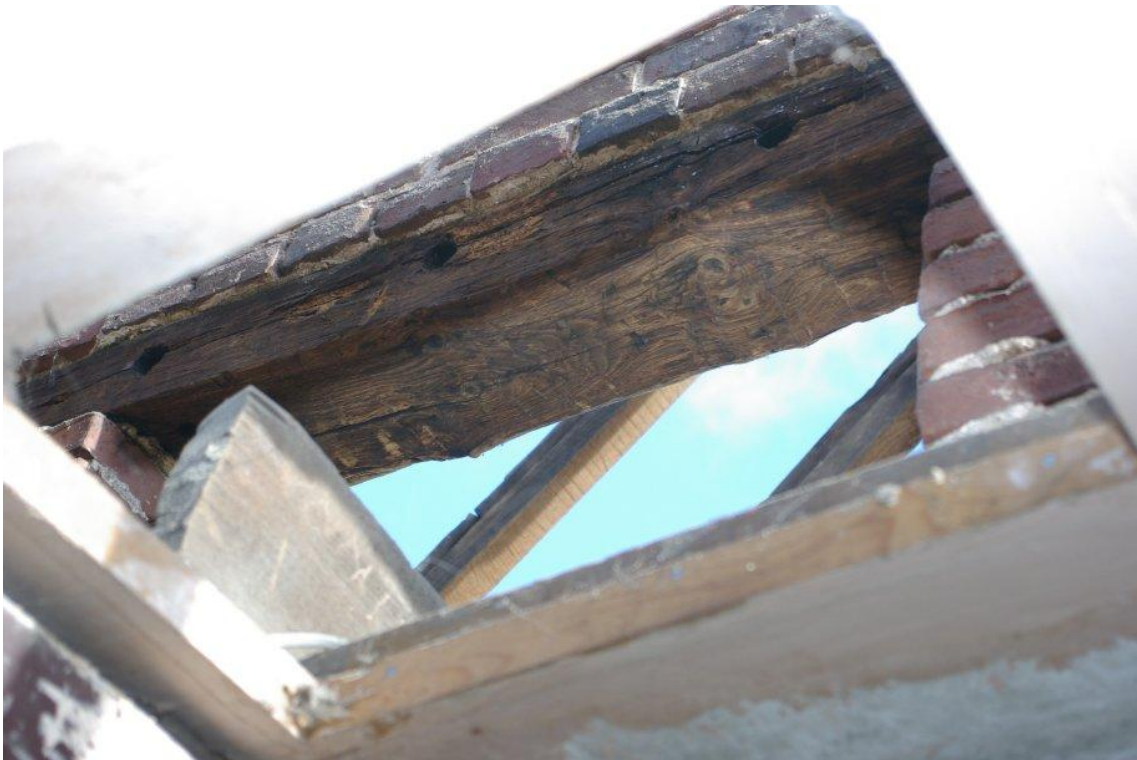
Figure 5 Limited view of re-used timber in attic space.
