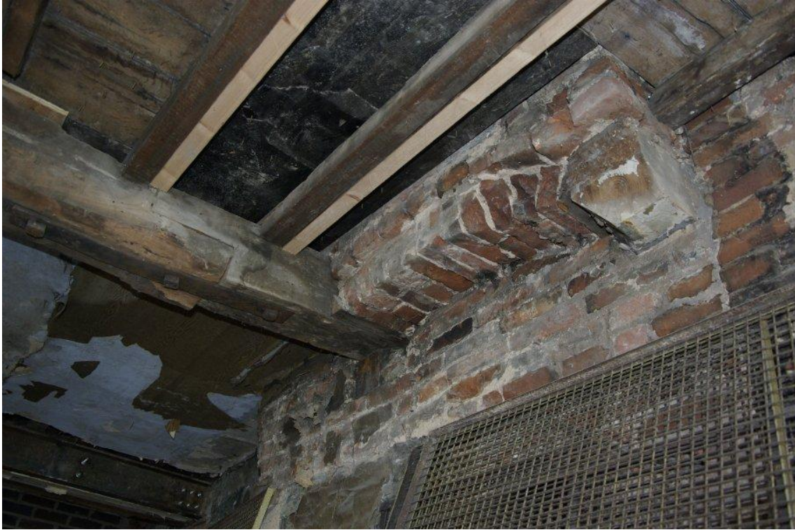
Figure 7 Inserted chamfered beam within G2.
