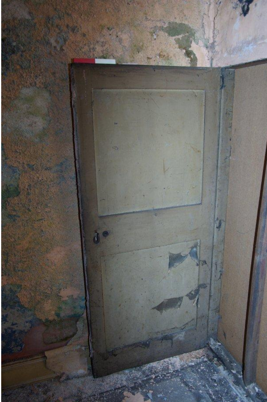
Figure 6 Original 2 panel door within F2.
