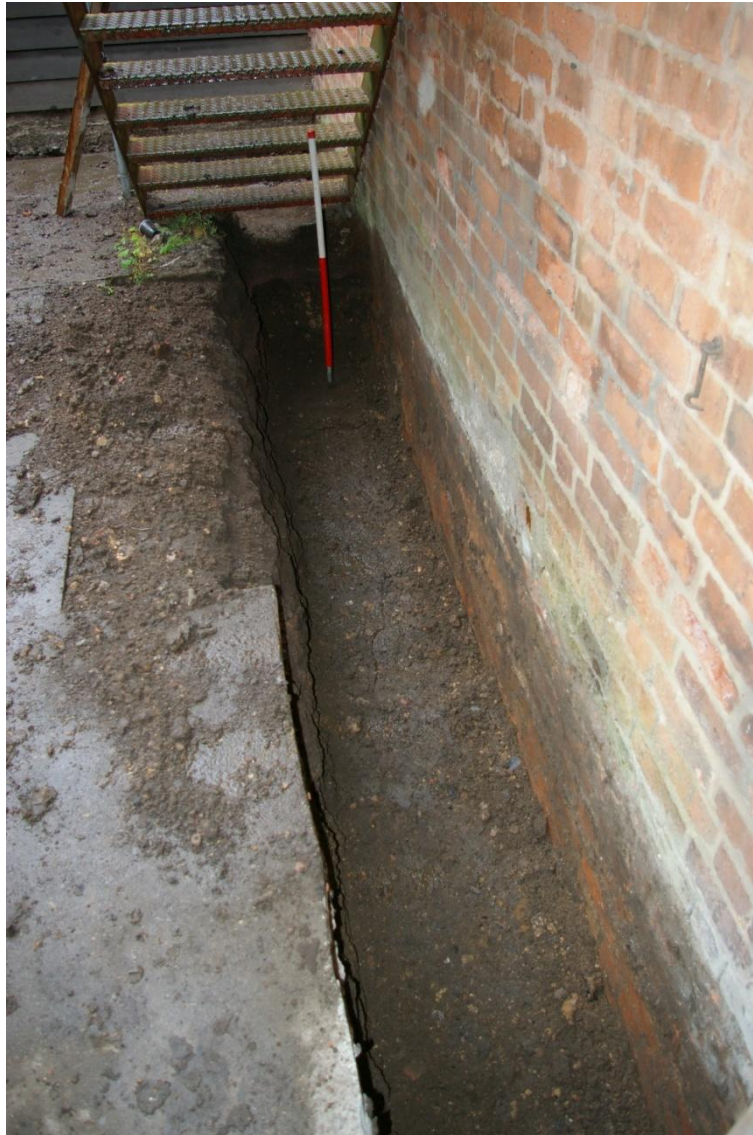
Figure 4 The west trench as excavated. Looking south.
