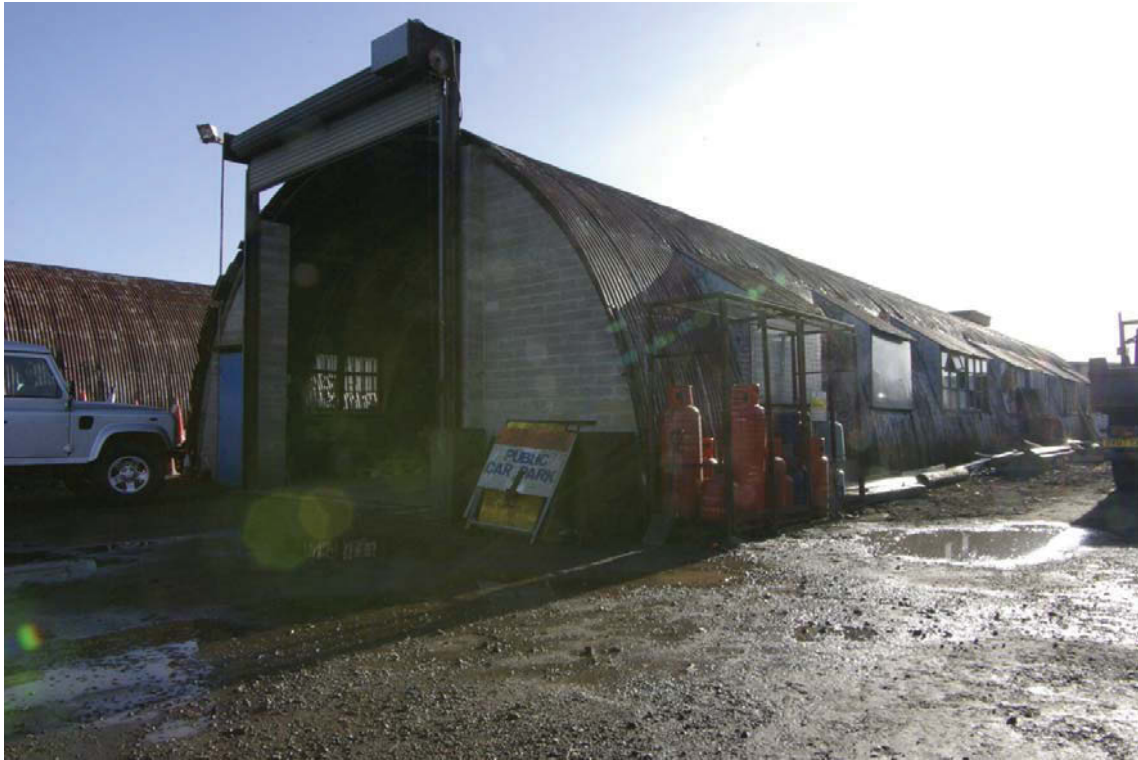
Figure 7: Building B (Looking South-east).
