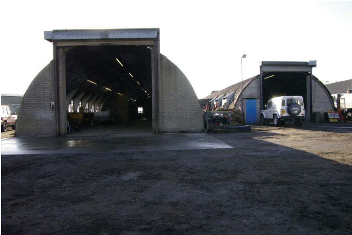
Figure 5: North facing elevations of the Nissan huts (Looking South).
