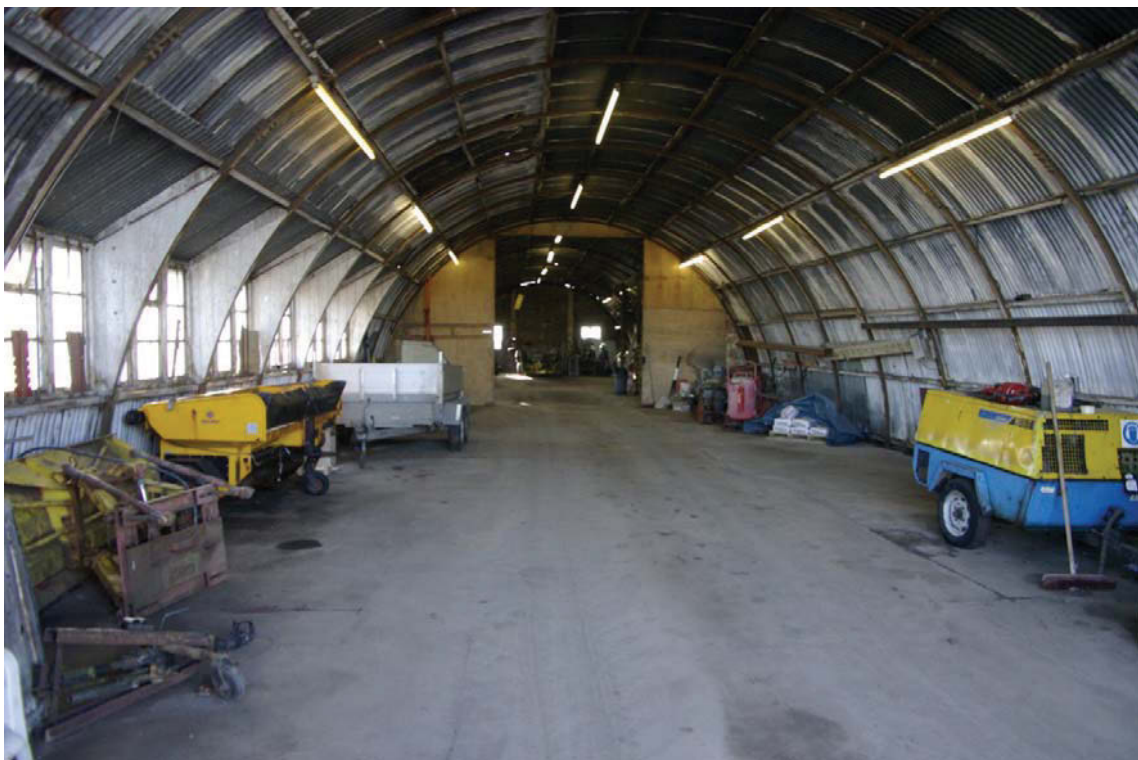
Figure 8: Building A, internal view (Looking South).
