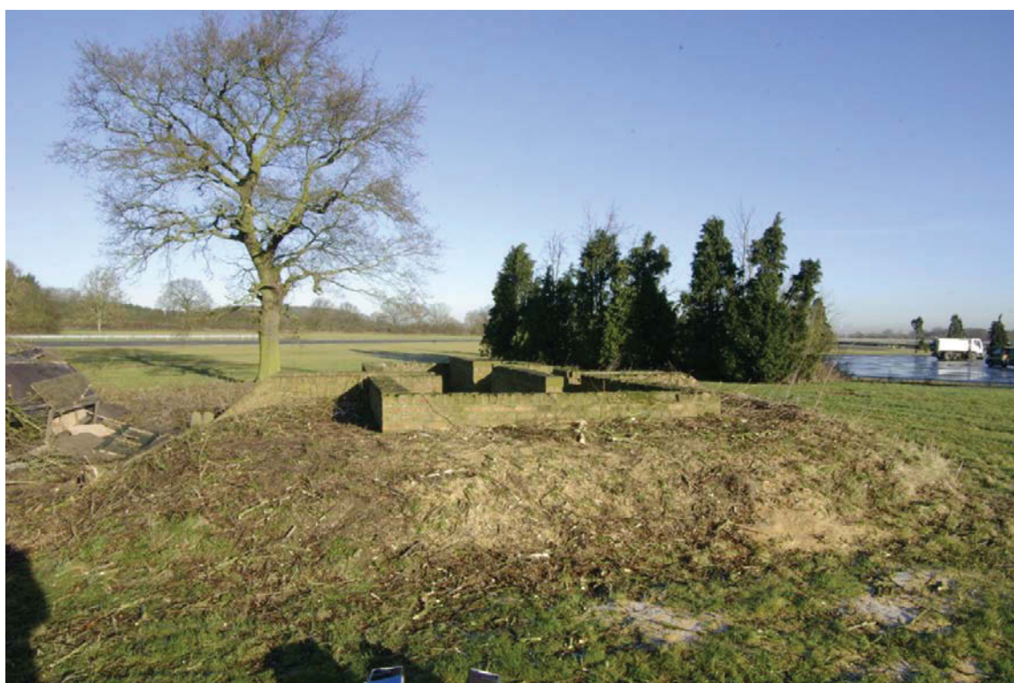
Figure 10: Blast Shelter (Looking North West).
