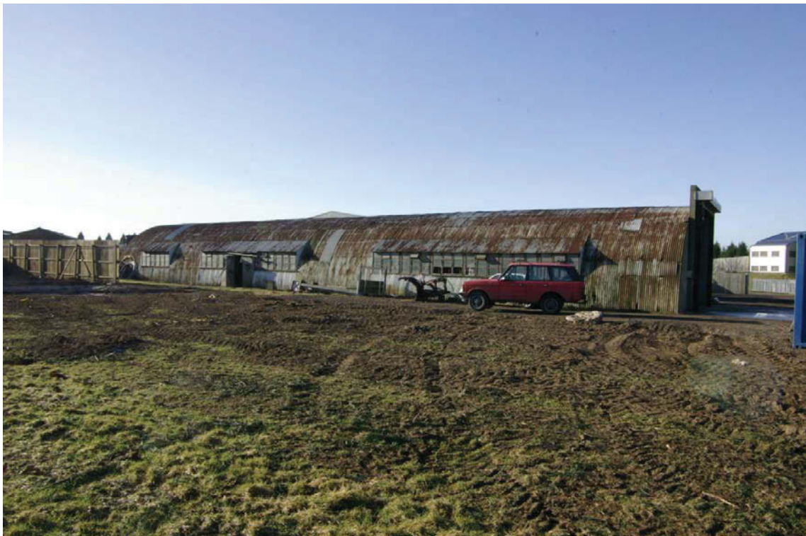
Figure 6: Building A (Looking West).
