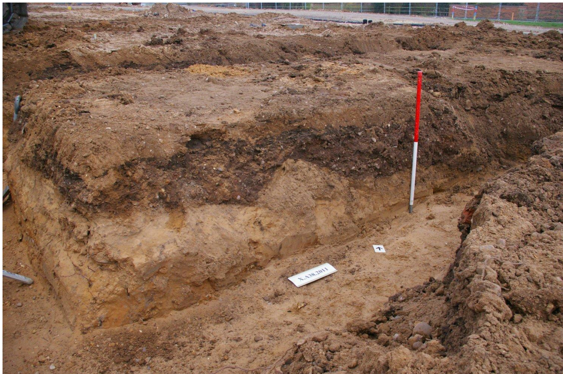
Figure 10 Evidence of quarrying seen within footings trenches.
