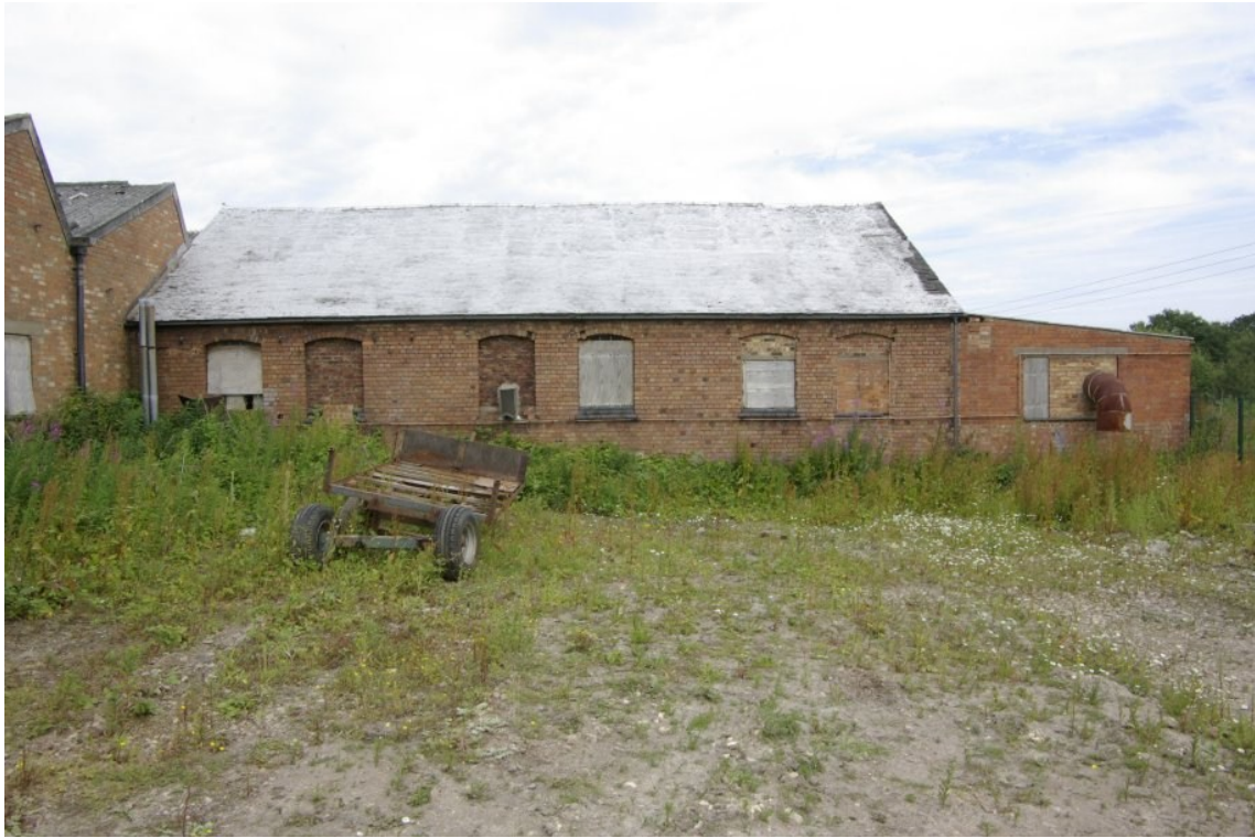
Figure 10 South-facing elevation of building 4.
