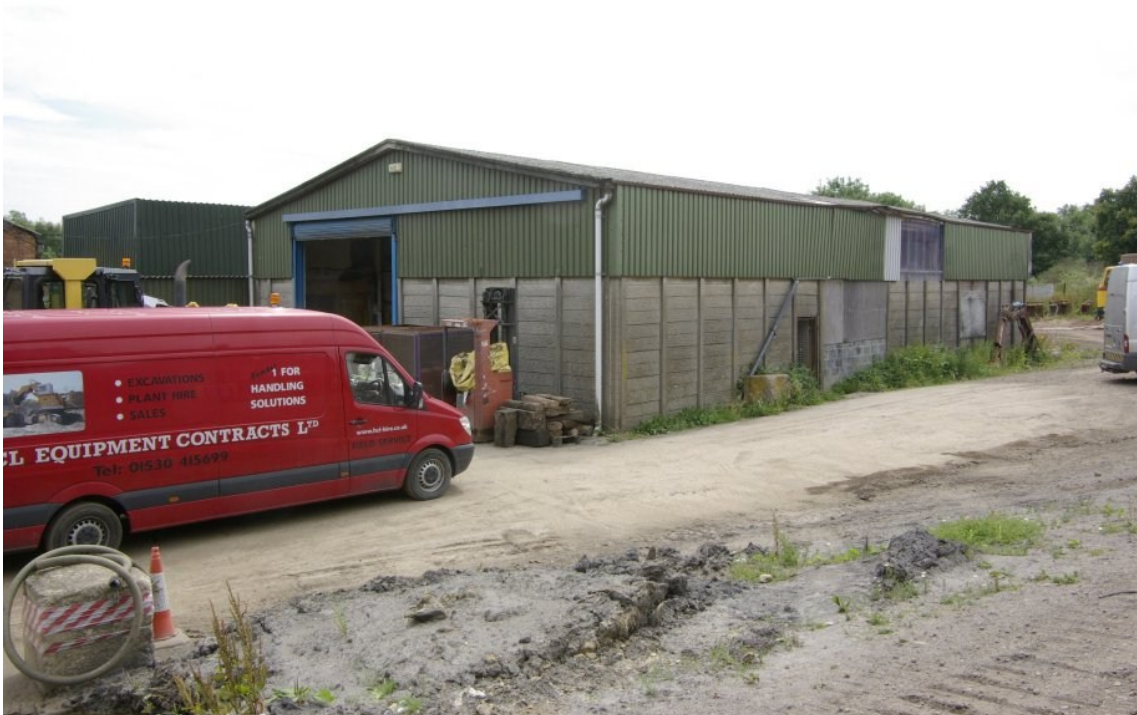
Figure 9 North- & west- facing elevations of building 5.
