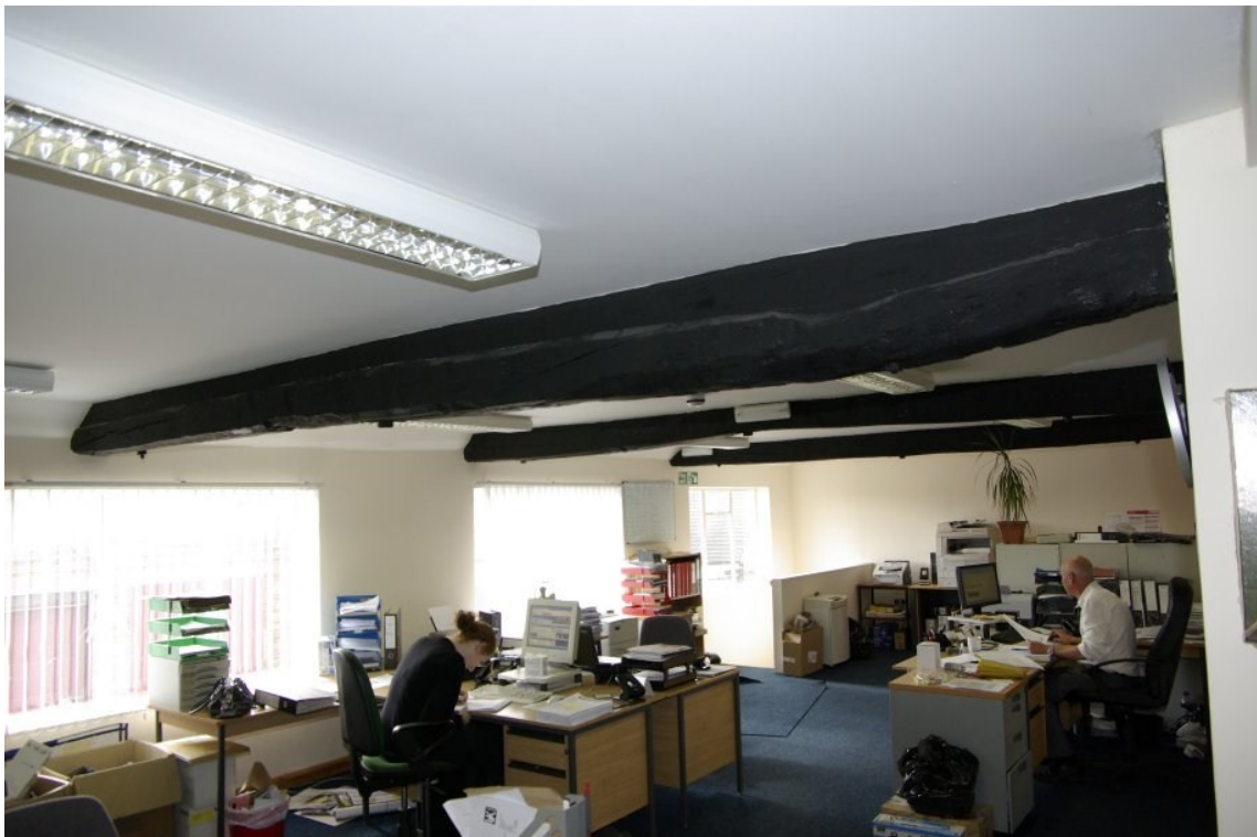
Figure 13 Partially exposed roof trusses within building 1a.
