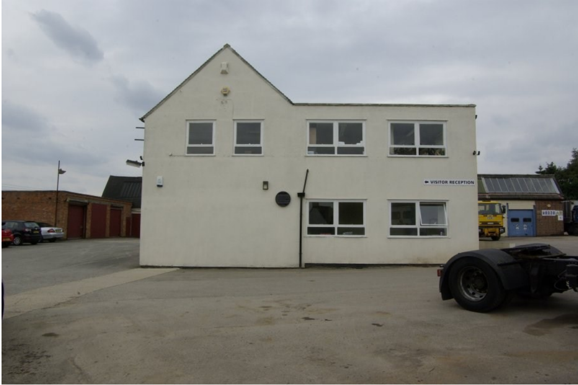
Figure 6 North-facing elevation of building 1.
