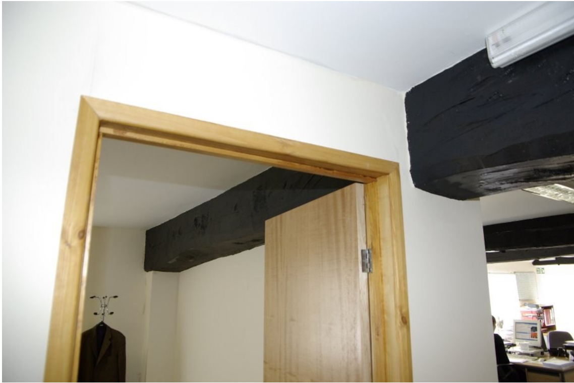
Figure 12 Partially exposed roof truss within building 1a.
