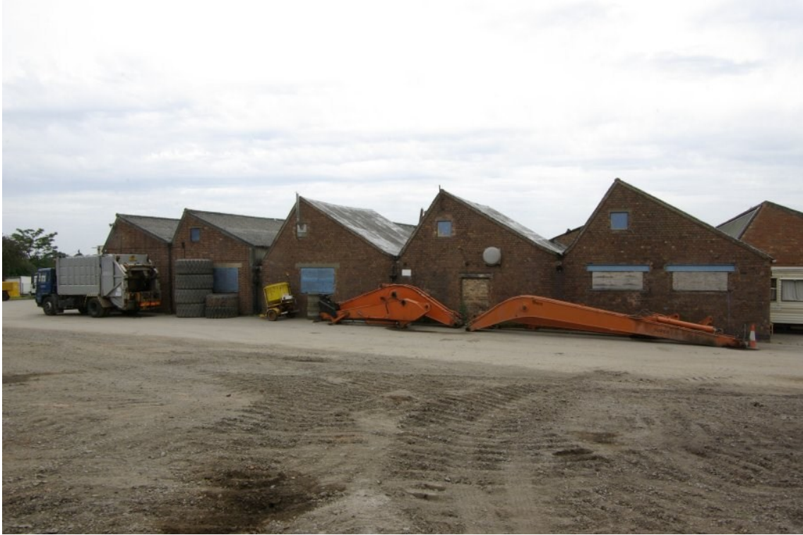
Figure 8 West-facing elevation of building 3.
