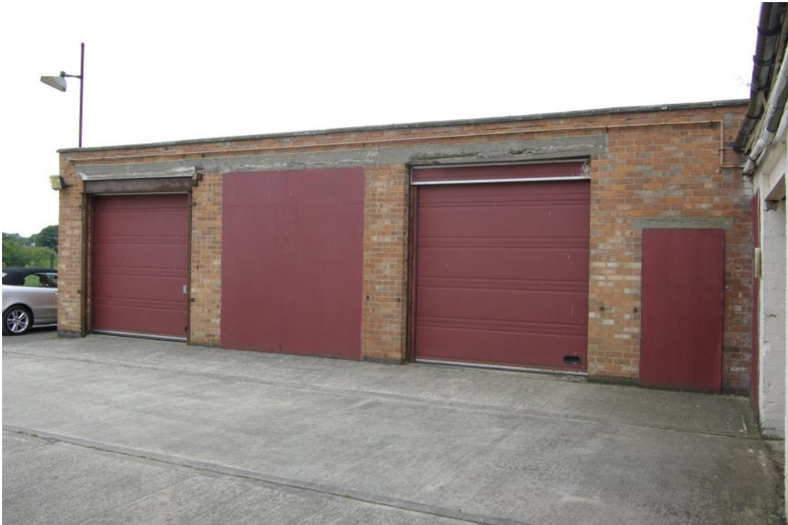
Figure 7 West-facing elevation of building 2.
