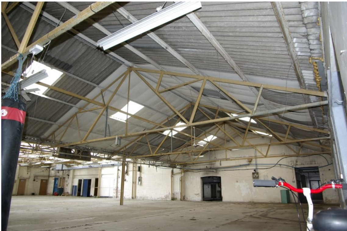
Figure 11 Building 3d, roof construction.
