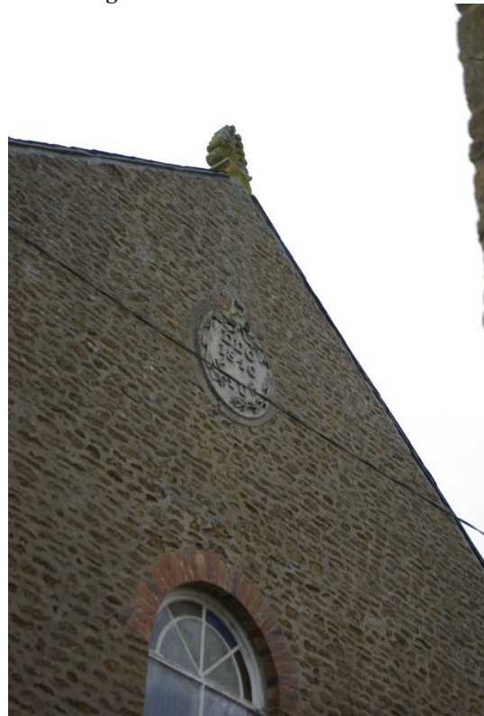
Figure 7 Date stone & finial, northern elevation.
