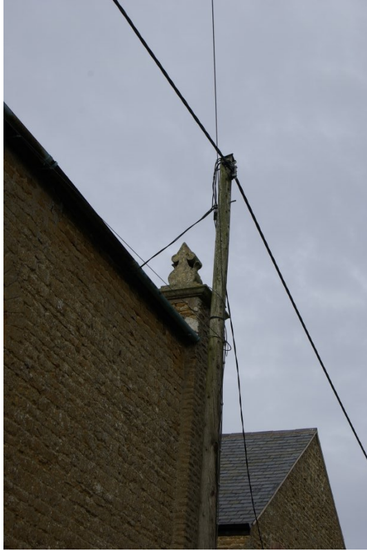
Figure 8 Pier cap, north east corner.
