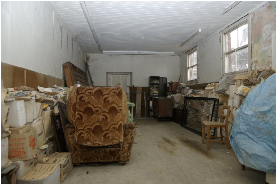
Figure 10 School room, internal, view east.
