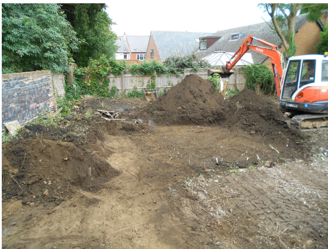
Figure 4: Garden soil removal in the northern (garden) area of the development site; view north
