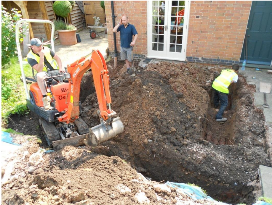
Figure 5: Machining of groundworks in progress; view southeast
