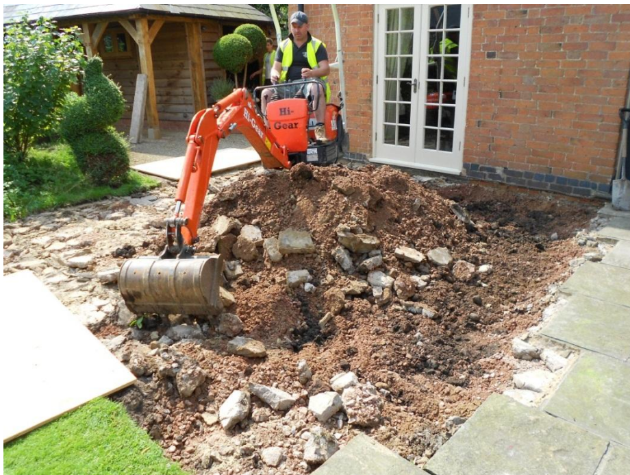
Figure 4: Machine removal of patio area in progress; view southeast
