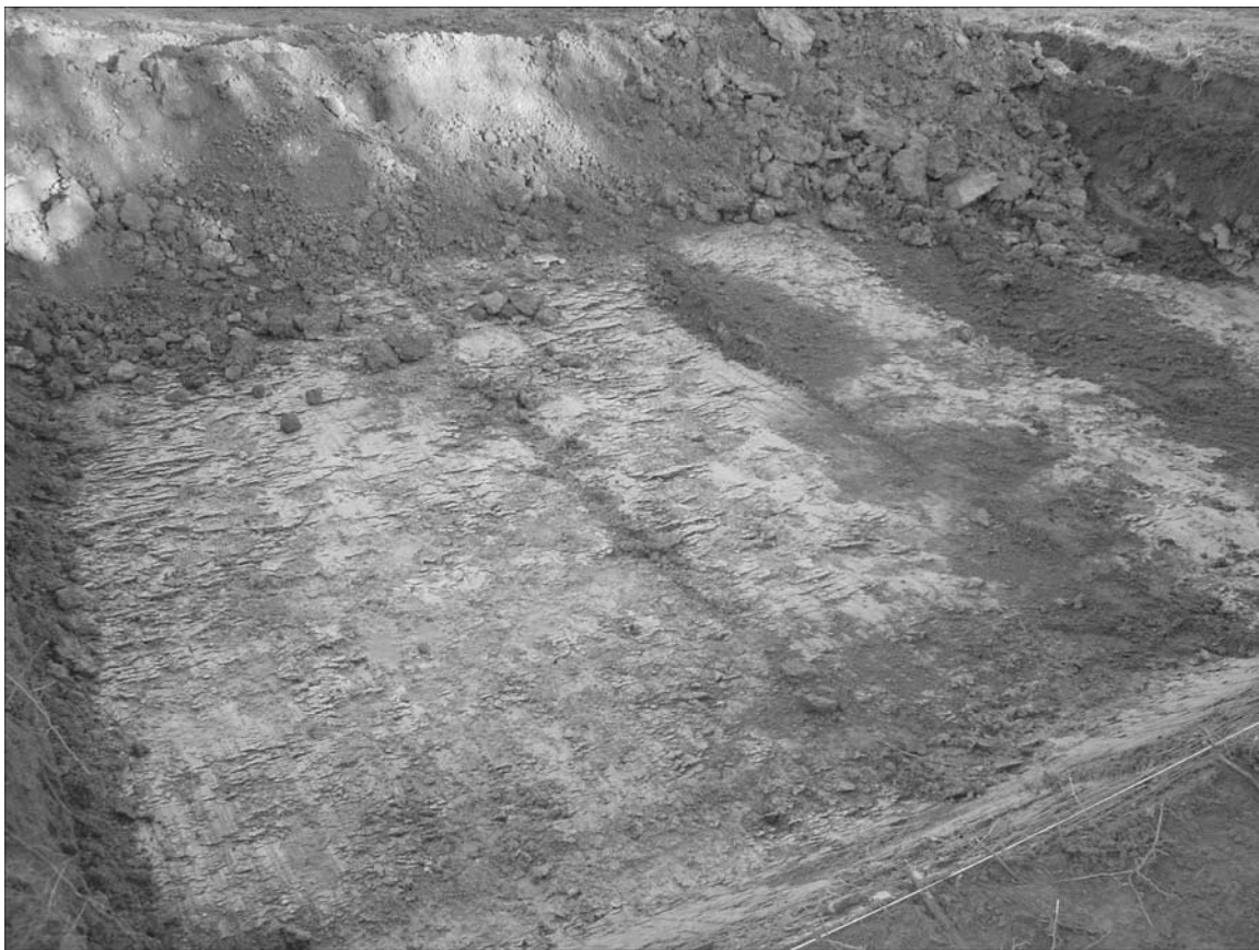
Fig. 4. Photograph of reed bed area once topsoil and subsoil have been stripped, facing north.
