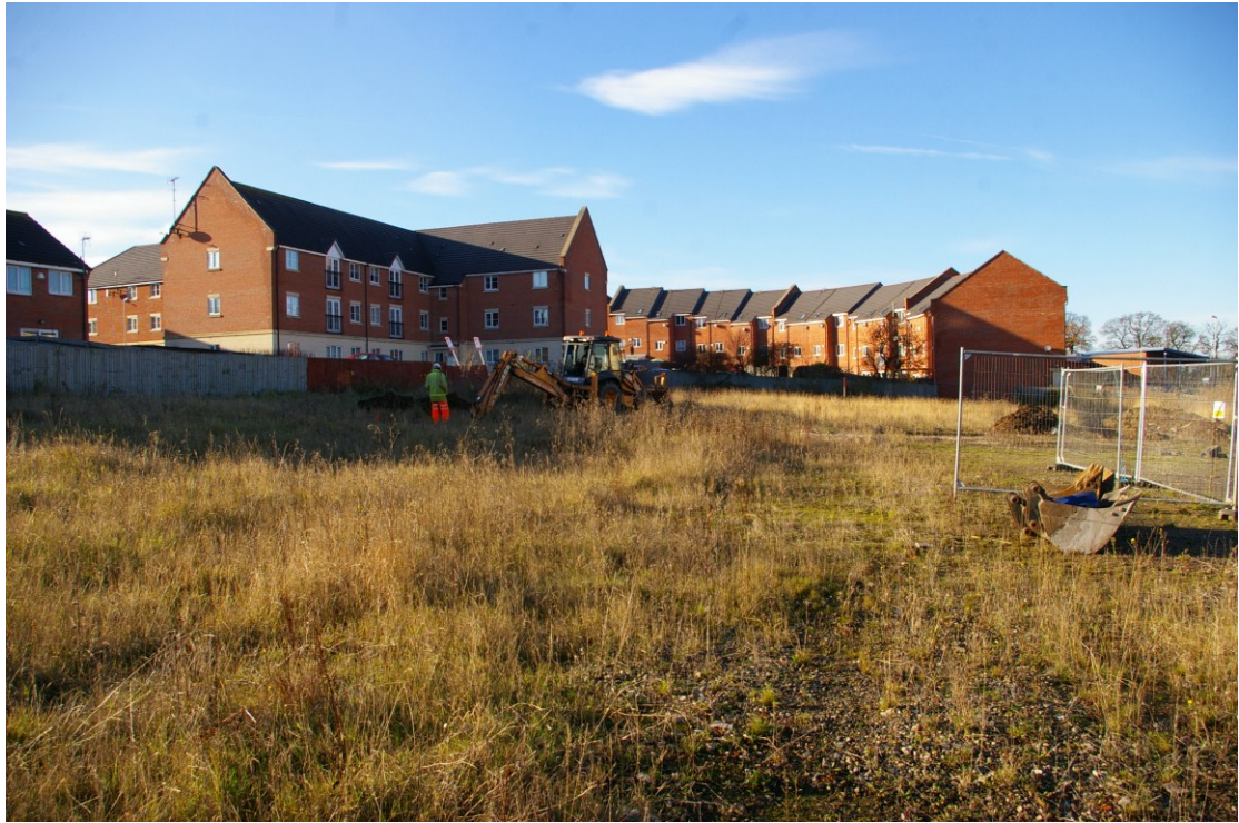
Plate 1: Work in progress on Trench 2, looking west
