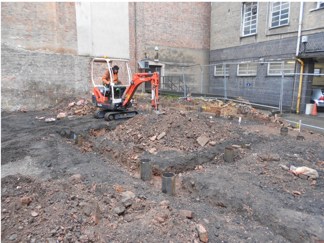
Figure 4: Working shot looking north-west, showing finished ground-beam trenches.
