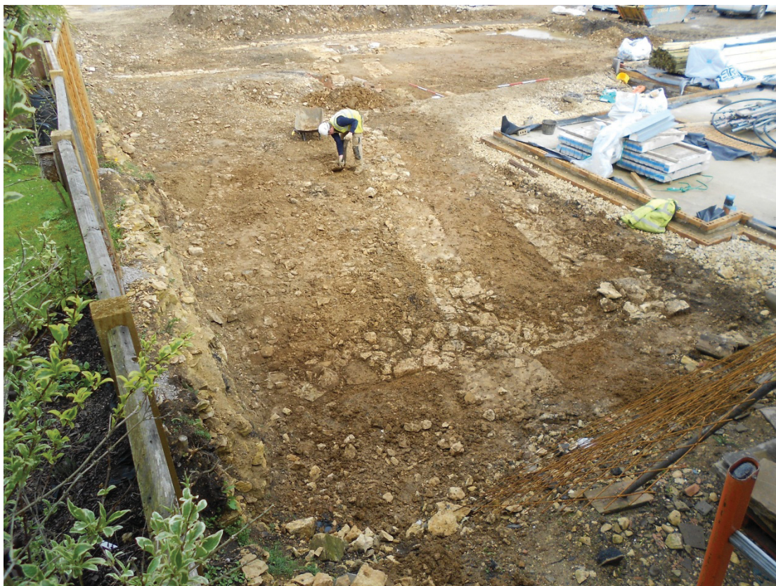
Figure 3: General view east across the area of excavation
