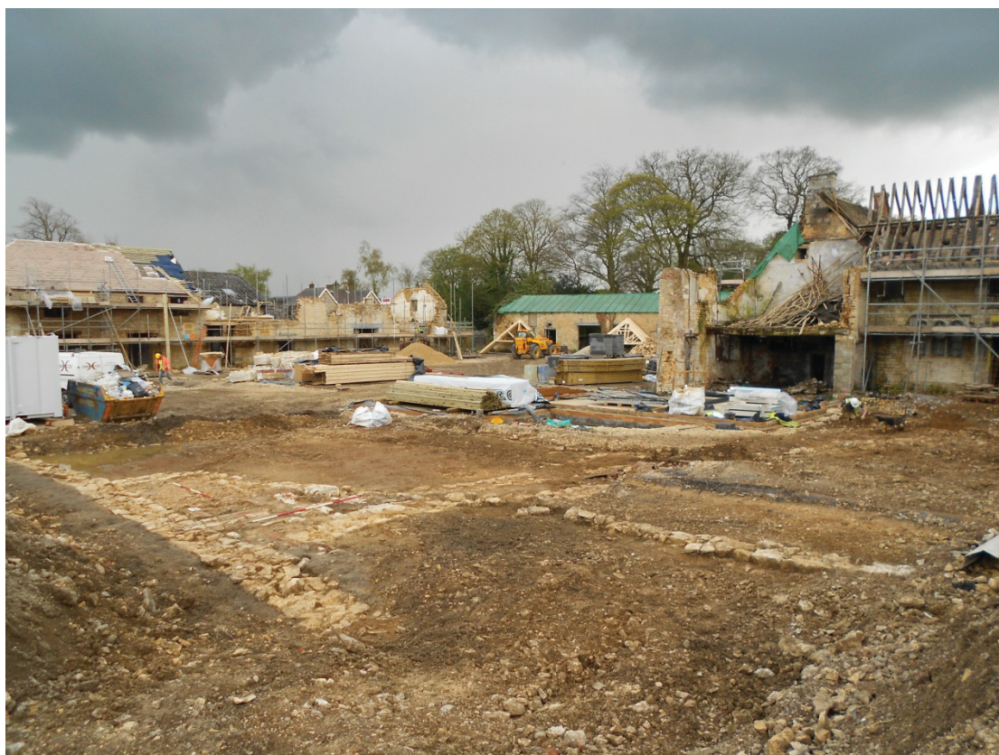
Figure 6: View south-west across excavation towards farm buildings
