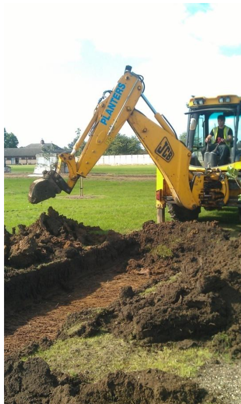
Figure 2: Machining in progress; view southwest
