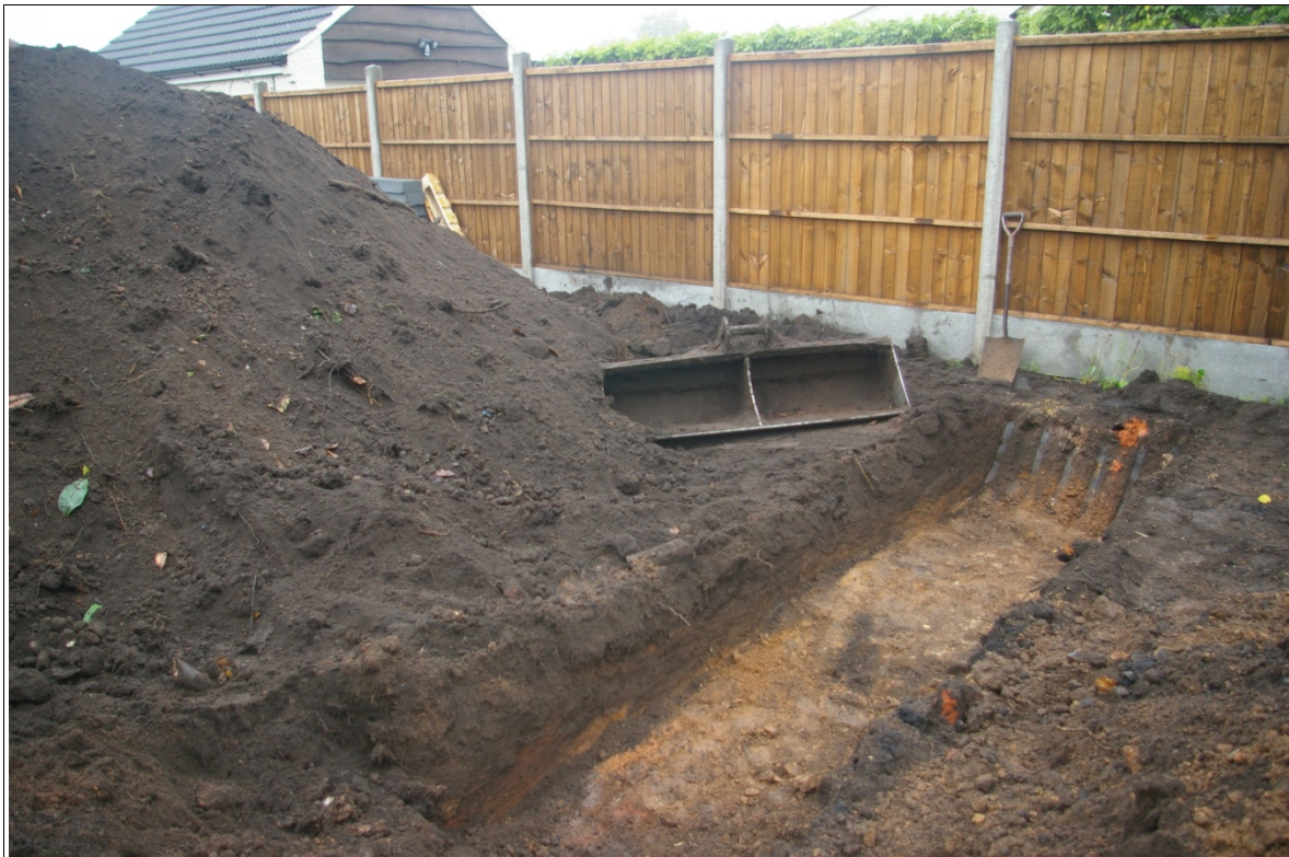
Figure 5. Trial hole at north-west of building footprint, shows sequence of modern deposits on to sandstone bedrock. Looking north-west
