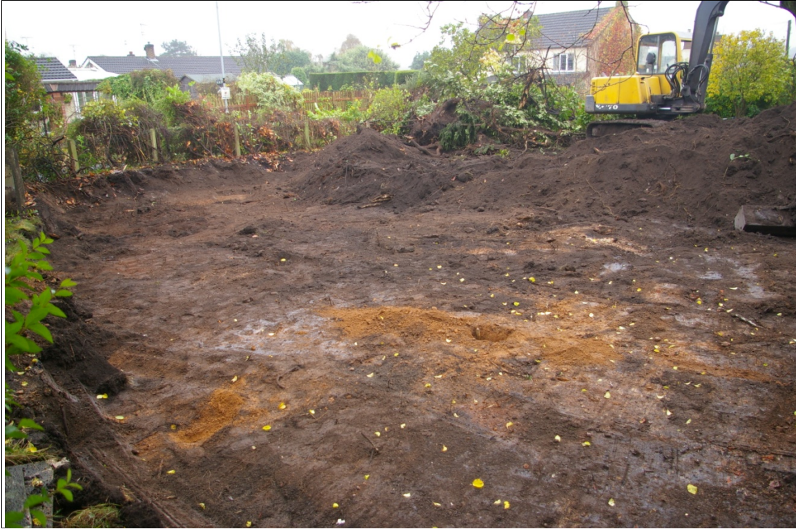
Figure 4. View from The Green frontage, looking south-west after reduced level dig. The lower, orangey material also produced modern material.
