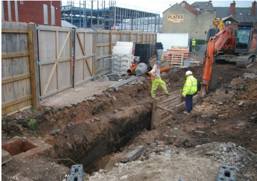
Fig. 6: Service trench adjacent to New Park Street (looking east)
