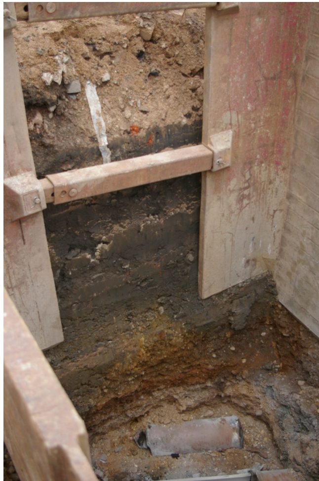
Fig. 5: ... Foxon Street (cont'd) Mineralised deposits adjacent to service trench (looking southwest)
