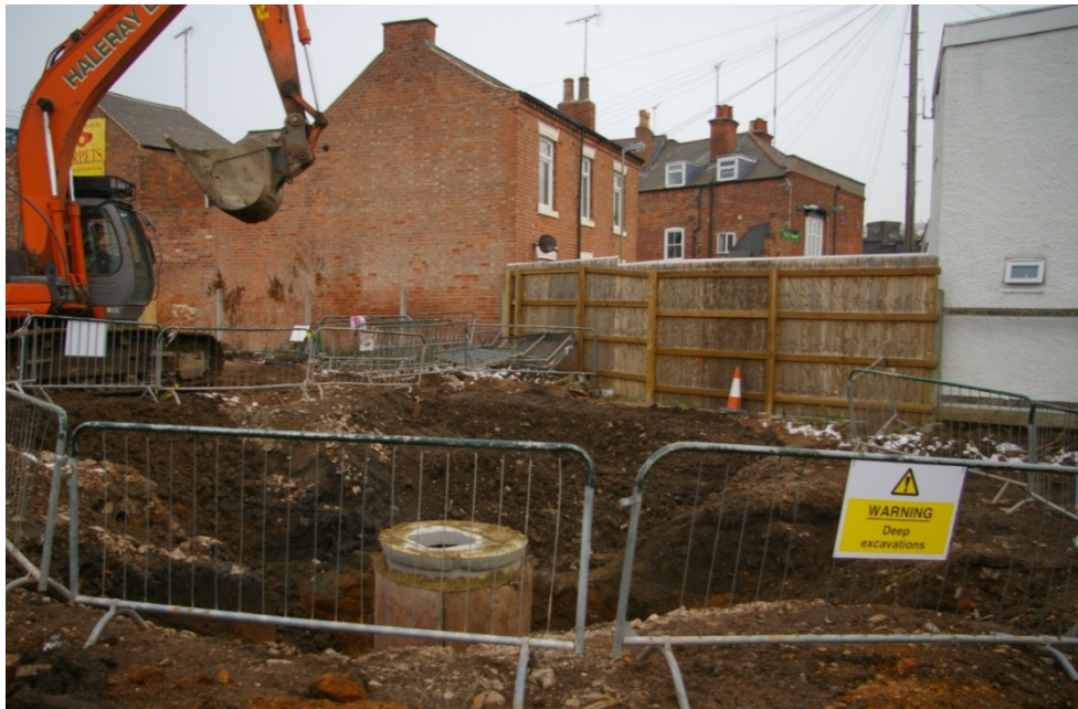
Fig. 7: New service works adjacent to Thorpe Street (looking east)
