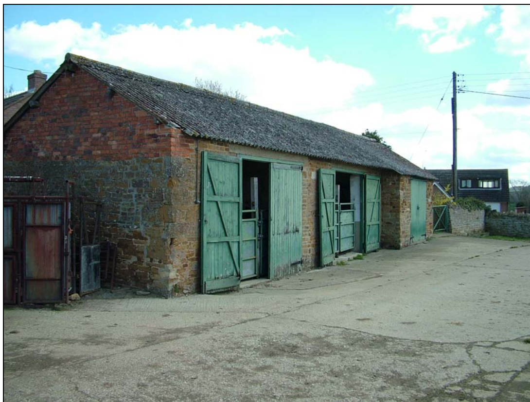
Plate 15: West face of stables looking south east
