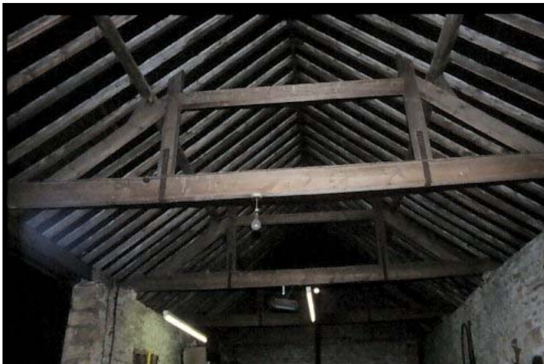
Plate 10: Internal roof structure of Barn C2
