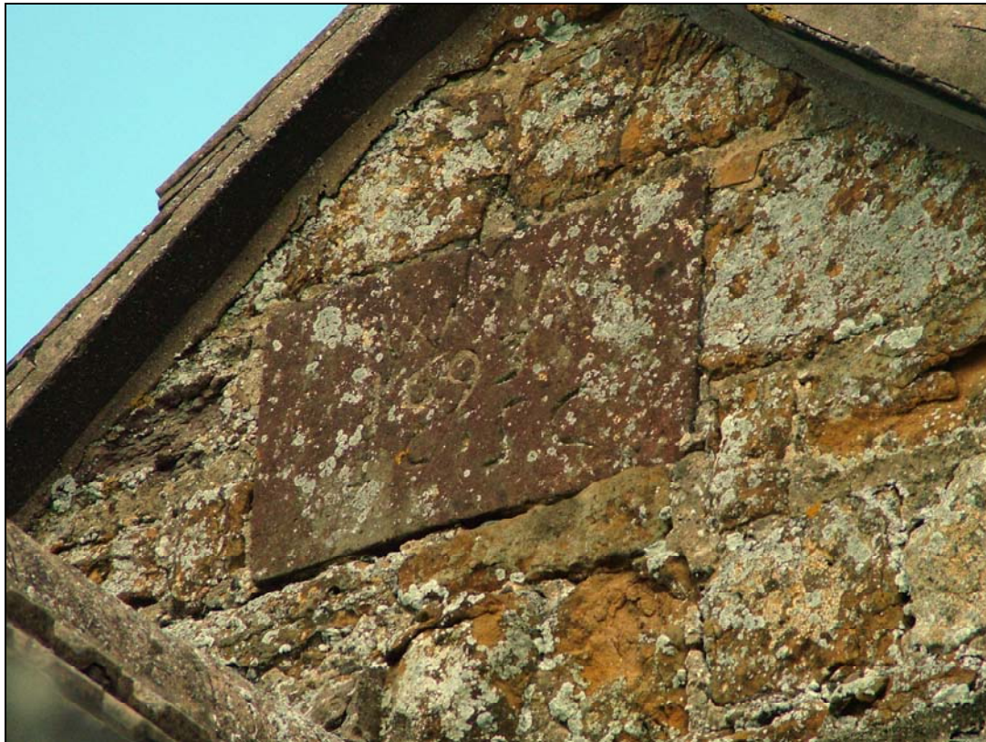
Plate 11: Ironstone face on east gable of barn C2
