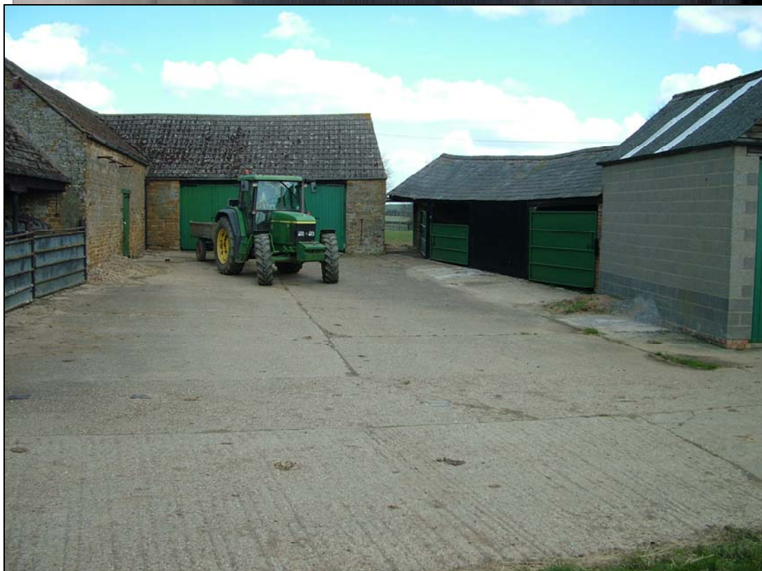
Plate 14: Courtyard buildings. West face of barn C3 and north face of barn C4
