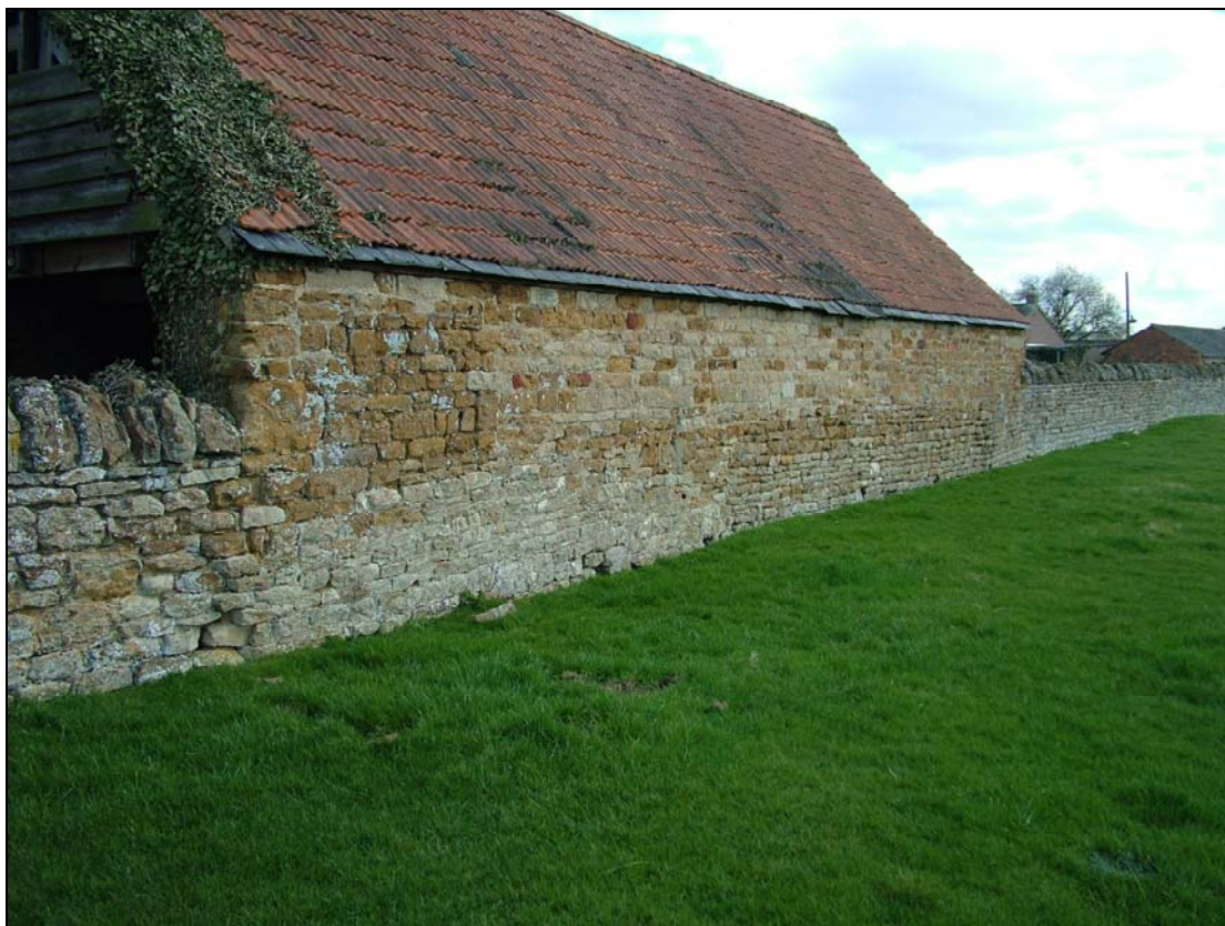
Plate 7: West wall of barn/ cart shed showing use of existing boundary wall, looking SE
