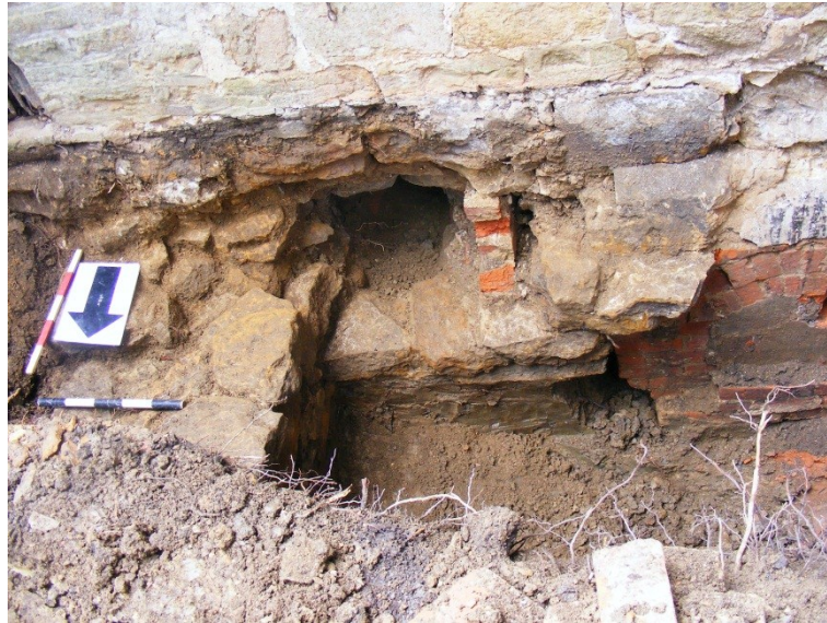
Figure 3: The possible buttress seen from above
