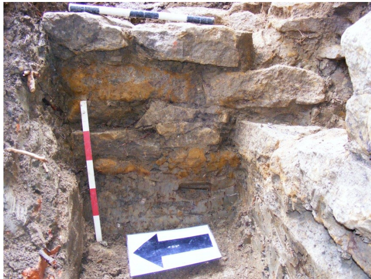
Figure 4: The possible buttress seen in elevation
