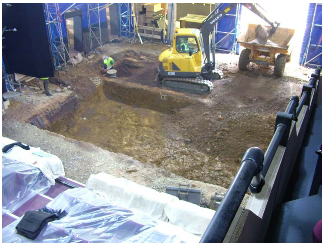
Figure 4: Work in progress on orchestra pit excavation, looking north west
