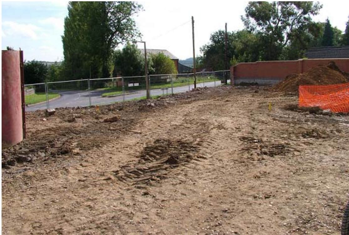
Plate 2: General view of site, looking south
