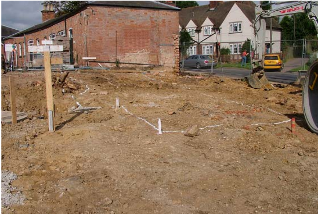
Plate 1: General view of site, looking north
