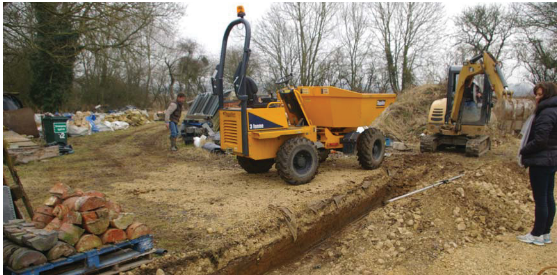
Plate 2: Work in progress, looking south-east
