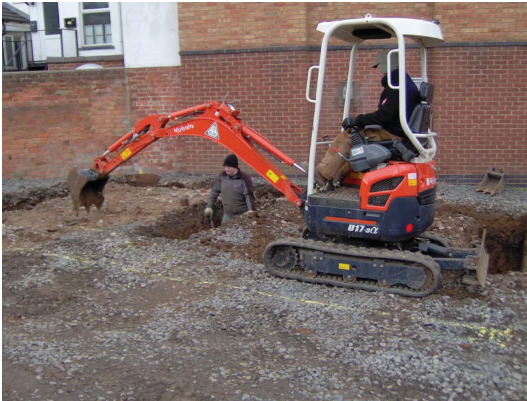
Plate 2: Work in progress on final trench, looking south-west
