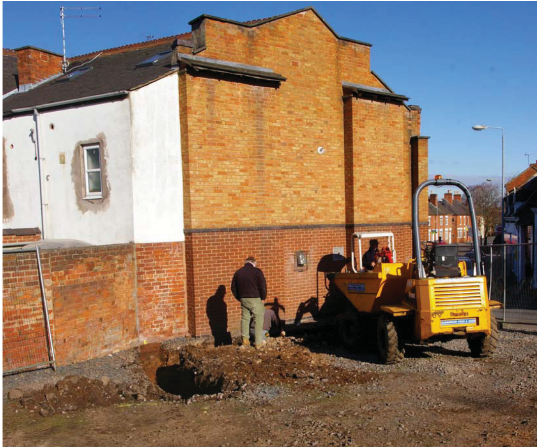
Plate 1: Work in progress against neighbouring property, looking west
