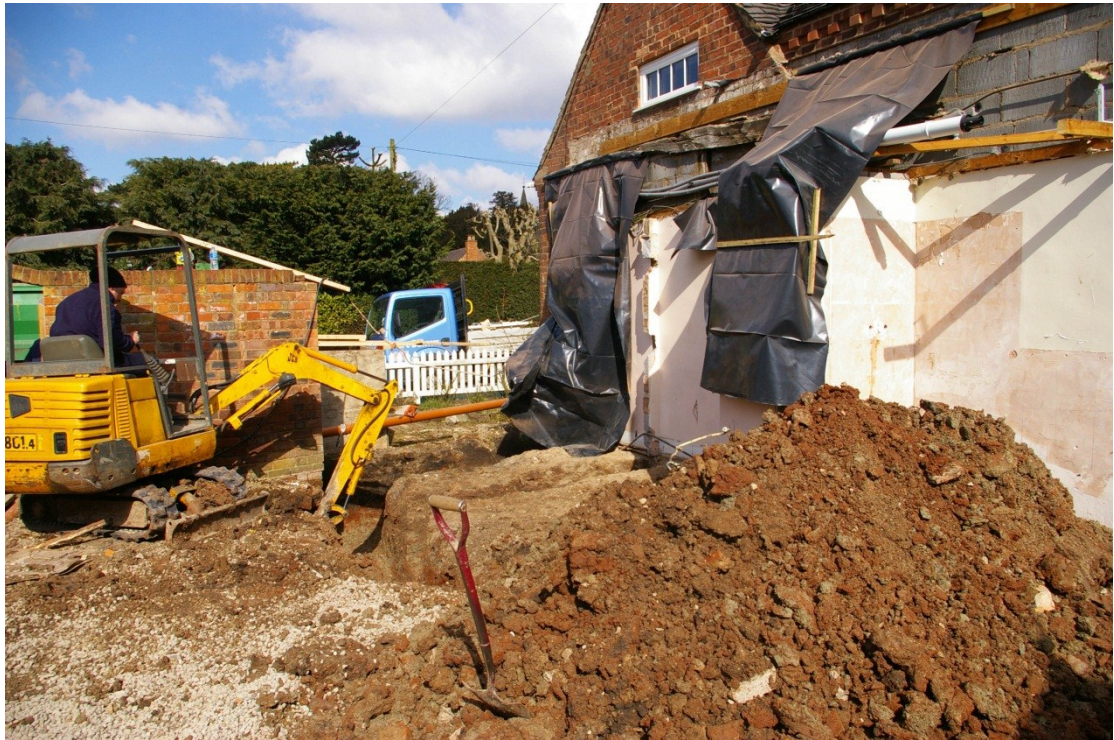
Plate 2: Work in progress, after demolition of previous extension, looking west
