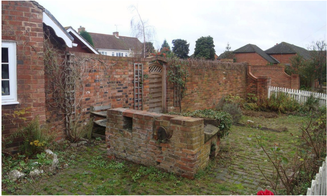
Plate 1: The furnace in the garden of The Forge, prior to demolition work. Looking south-east
