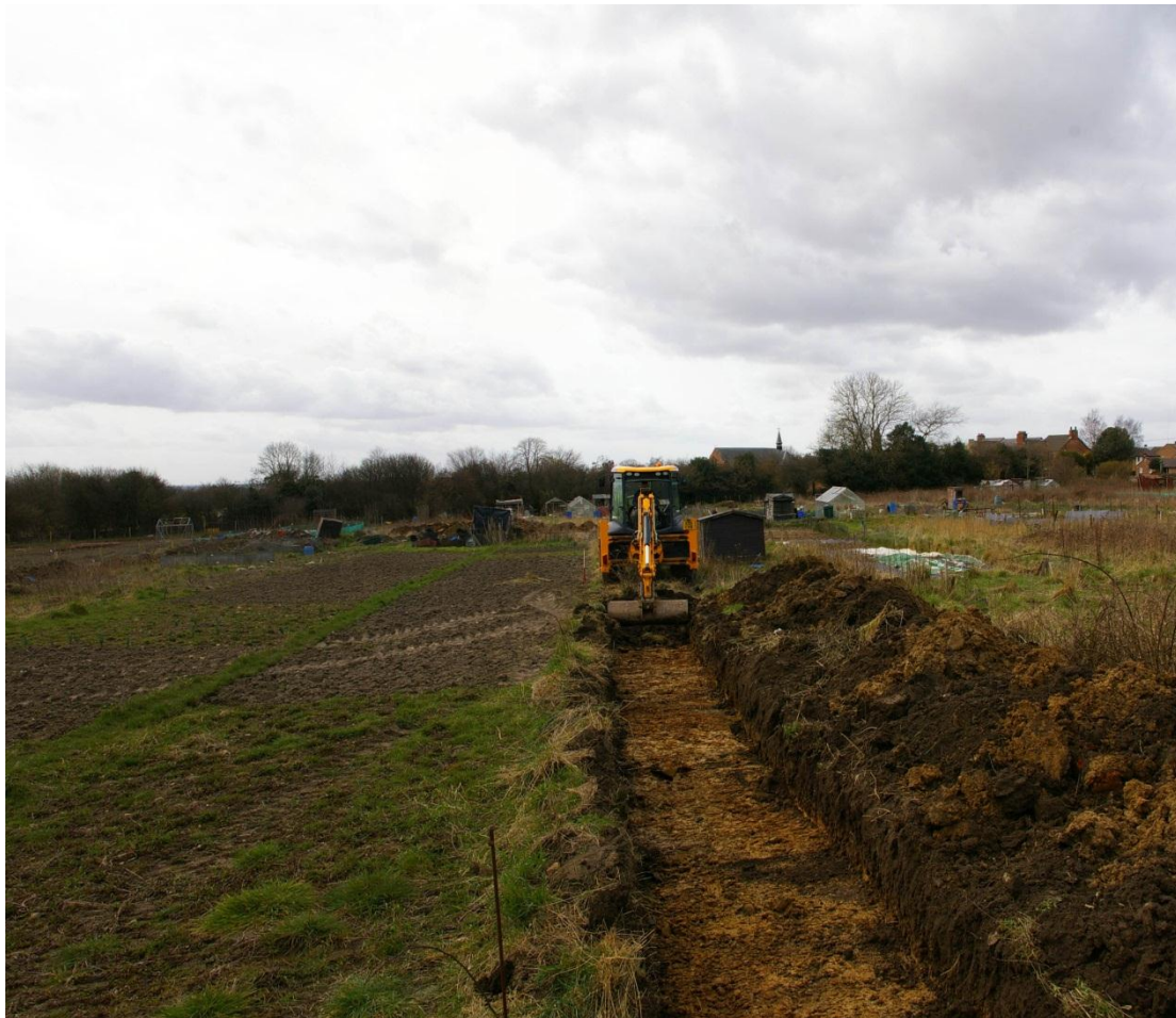
Plate 1: Work in progress on Trench 12, looking south-west
