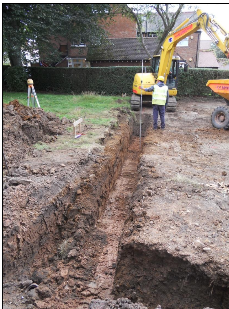
Figure 3 Machine excavating foundation trenches
