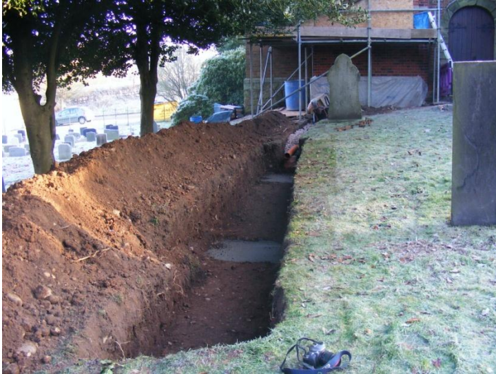
Figure 3: View of the soakaway and drainage trench (looking east)
