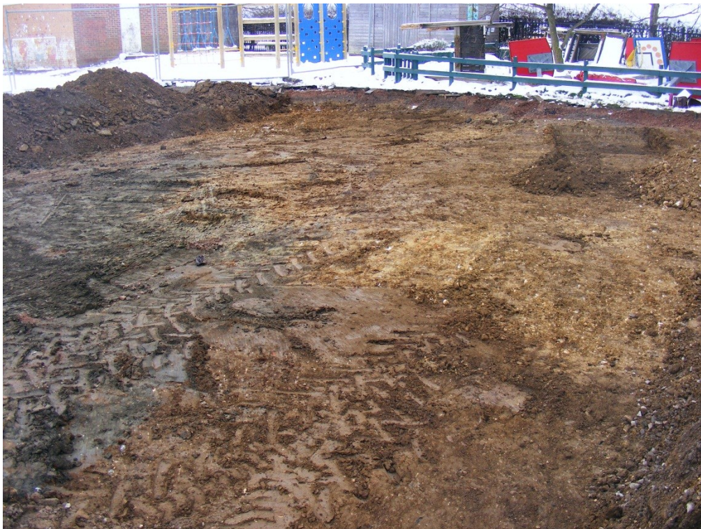
Figure 4: North-facing view over stripped area, showing buried topsoil (right) and buried turf (left) in the foreground and re-deposited subsoil towards the back
