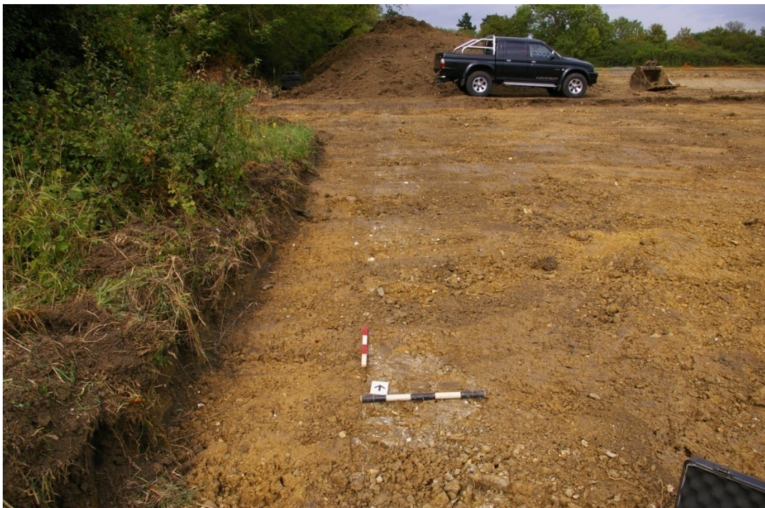
Figure 3: Example of the stripped surface, showing a service trench aligned NNE-SSW
