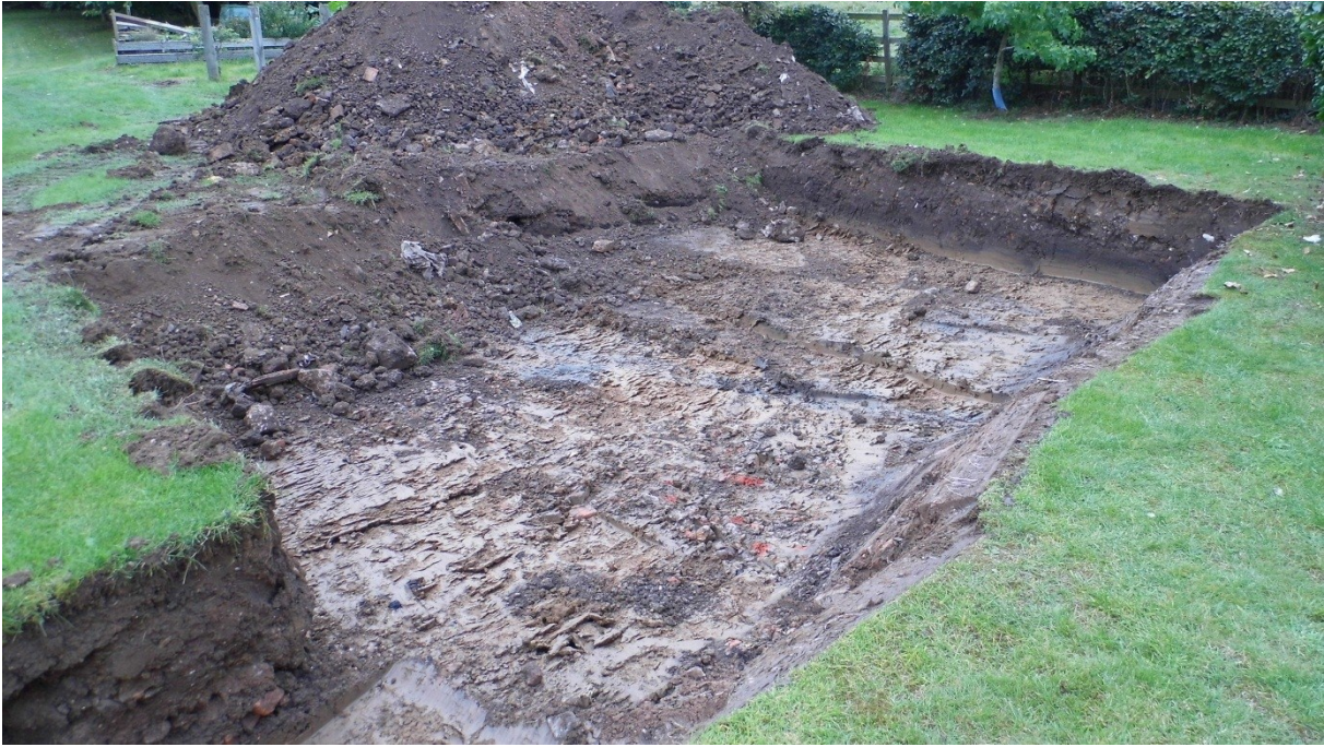
Figure 2: the southern half of the building footprint, looking south-east
