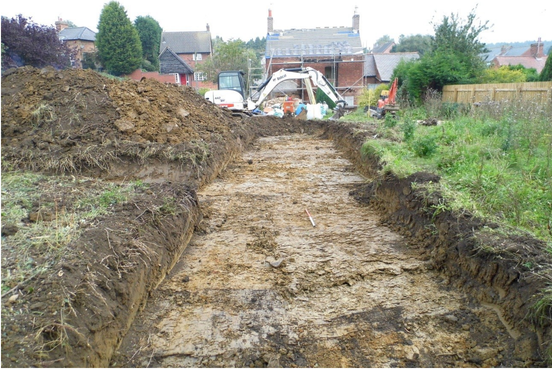
Figure 3: The stripped building footprint in Plot B, looking north-east
