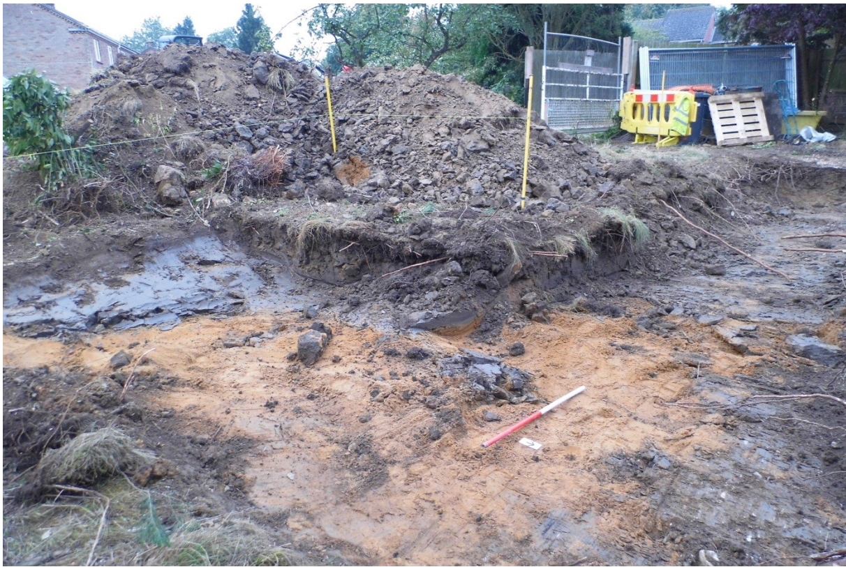
Figure 2: The stripped building footprint in Plot A, looking south-west
