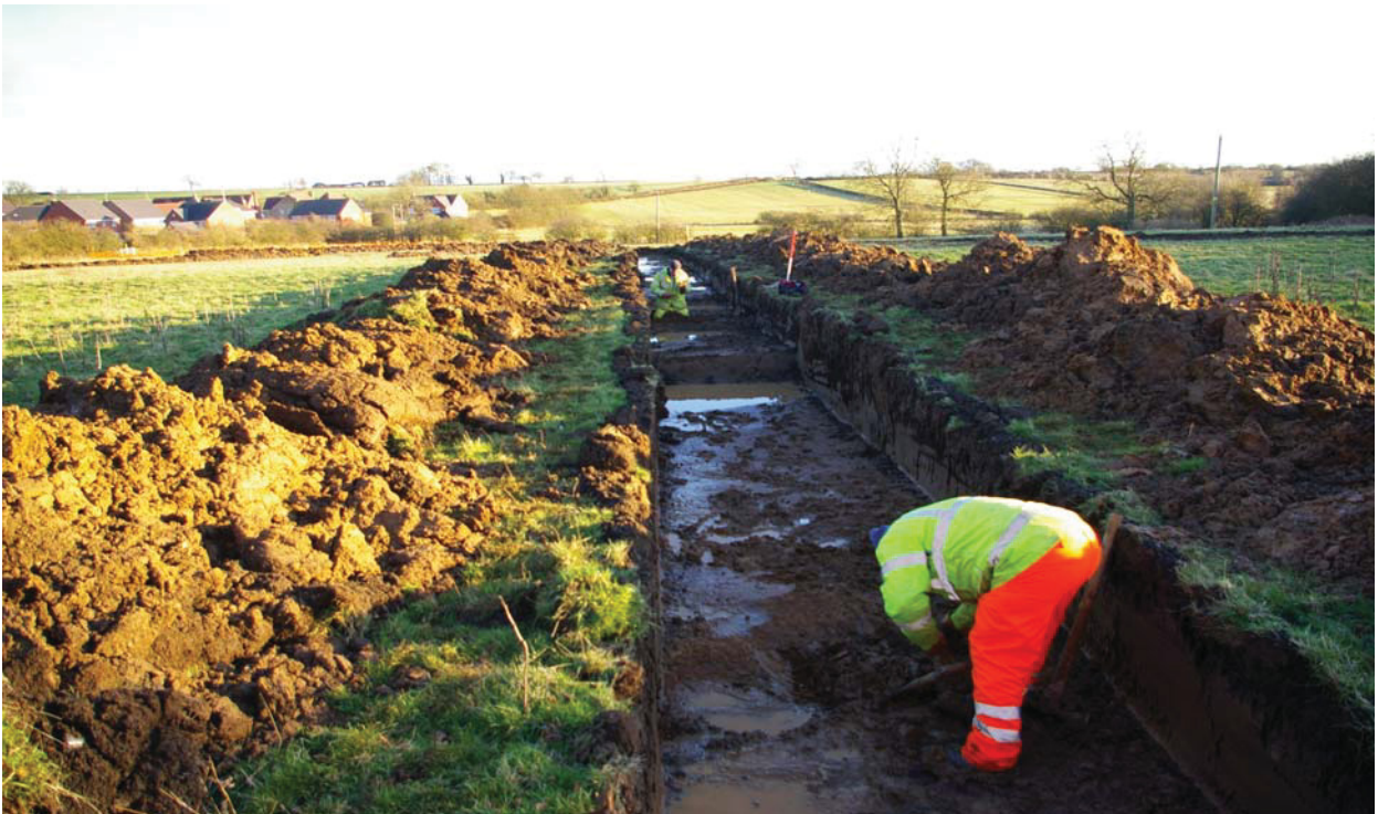
Plate 2: Work in progress on Trench 2
