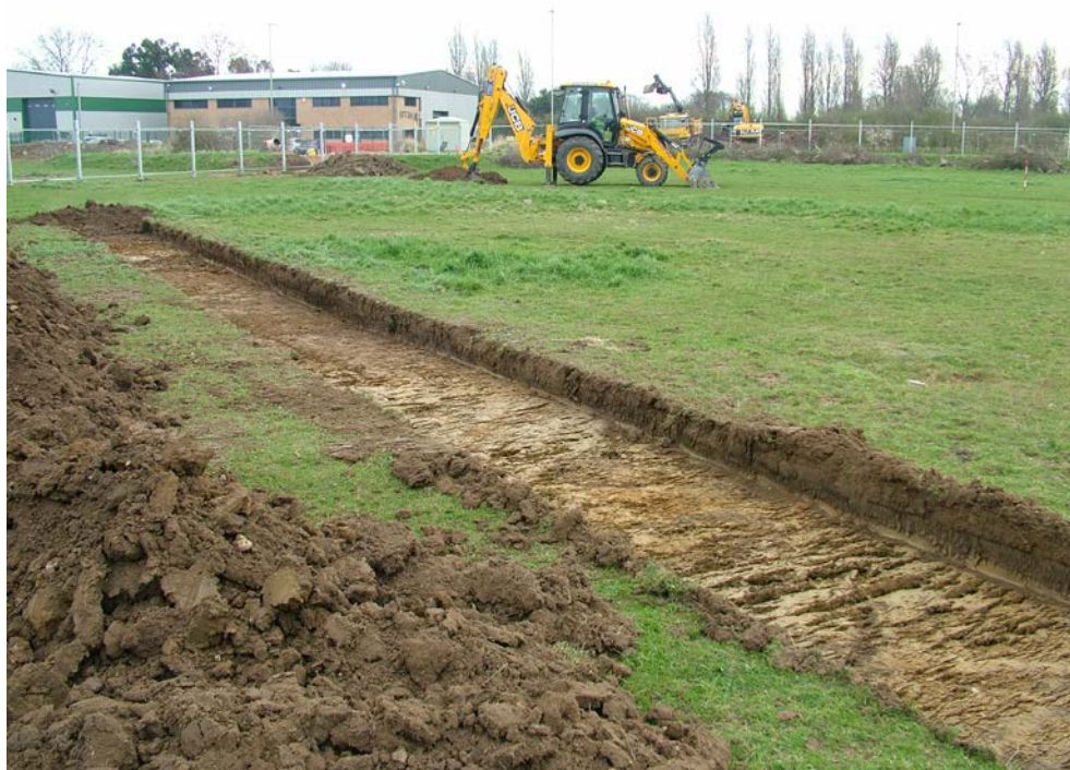
Plate 1: Work in progress on Trench 02, looking east
